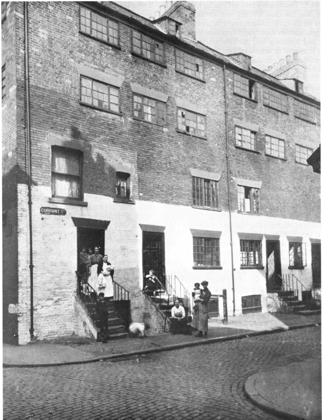
PLATE 3: Housing in Currant Street: five stories and a garret; in 1919 two floors have 'framework knitters' windows, though that does not mean there were frames behind all of them.
