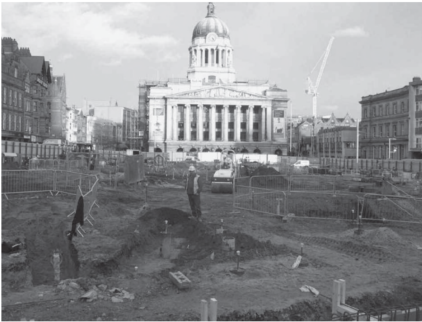
PLATE 1: General view of the wall after excavation looking east.
