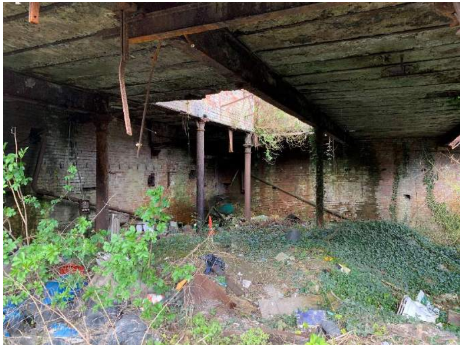
Plate 22: Interior of Building 3 looking west from exterior
