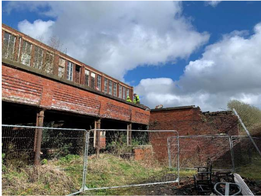
Plate 17: East end of southeast elevation of Building 2 looking north
