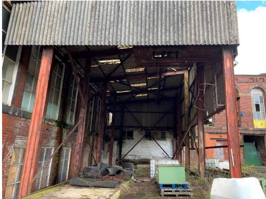
Plate 10: Southwest elevation of Building 1 looking northeast
