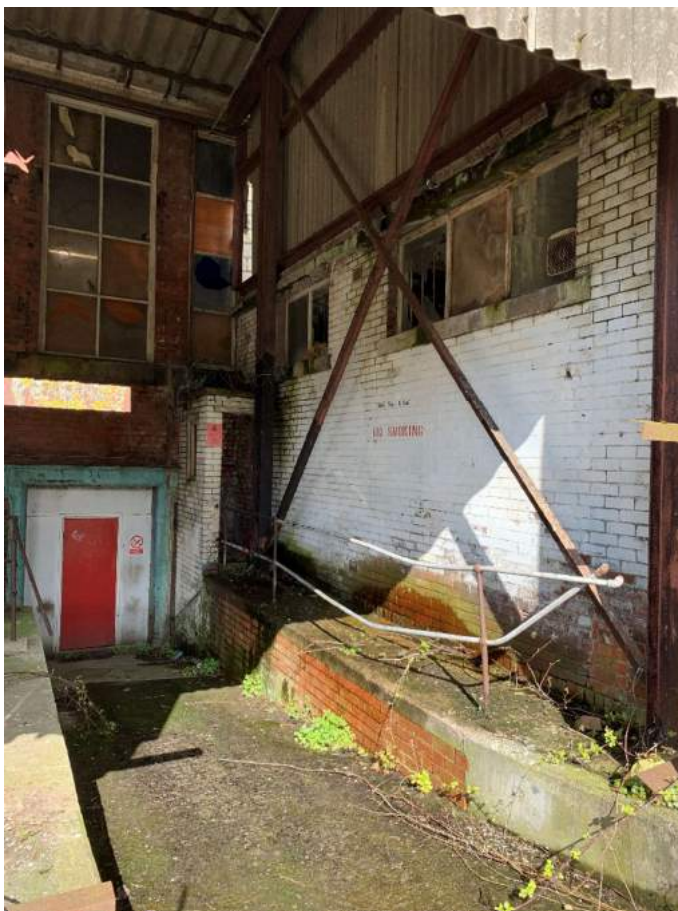
Plate 11: Interior north corner of Building 1 looking north from exterior
