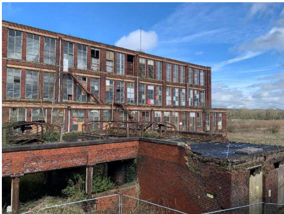
Plate 18: East end of southeast elevation and roof of Building 2 looking north
