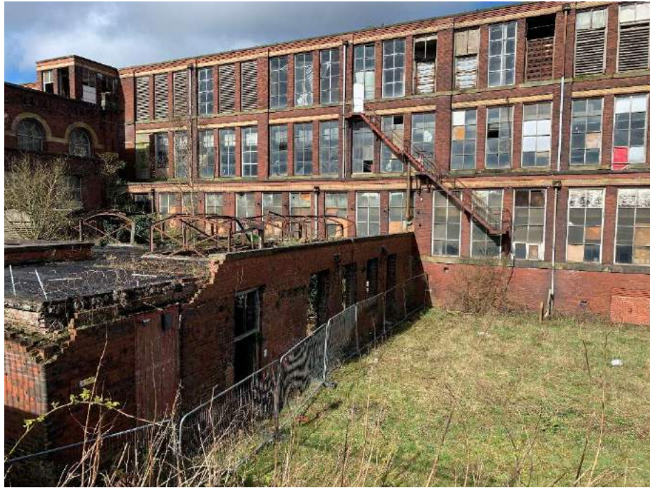
Plate 19: Northeast elevation and roof of Building 2 looking southwest
