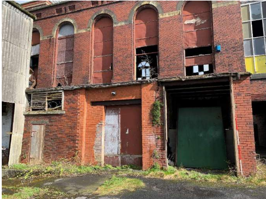
Plate 13: Southwest elevation of Building 2 looking northeast
