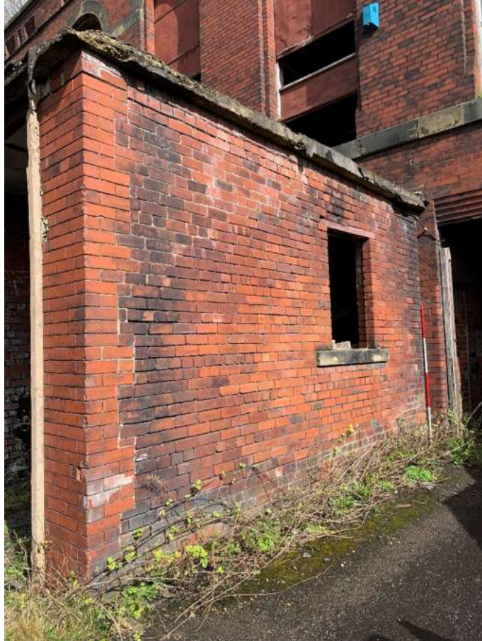
Plate 15: Southeast elevation of building 2 looking north
