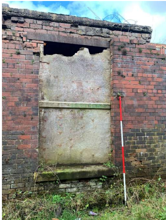
Plate 20: East window opening in southwest elevation of L-shaped popout of Building 2
