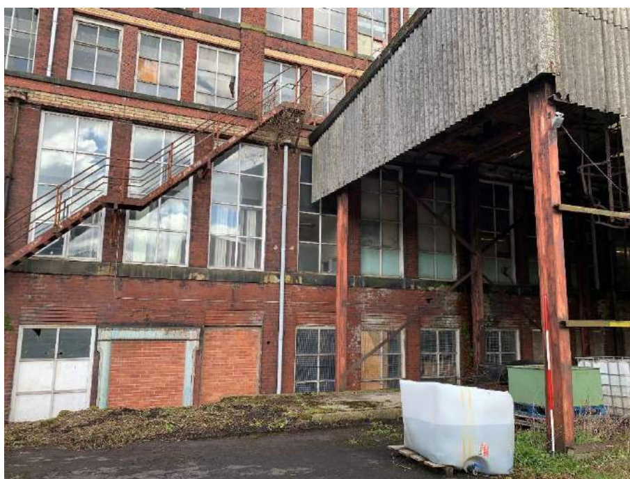
Plate 12: Southwest elevation of Building 1 looking north
