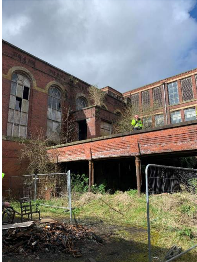
Plate 16: West end of southeast elevation of Building 3 looking west
