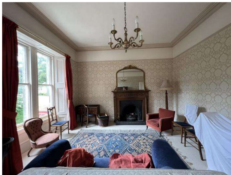
Plate 11: Fireplace, window panelling, and decorative cornicing in drawing room on first floor, looking north (RKA Architectural Design)
