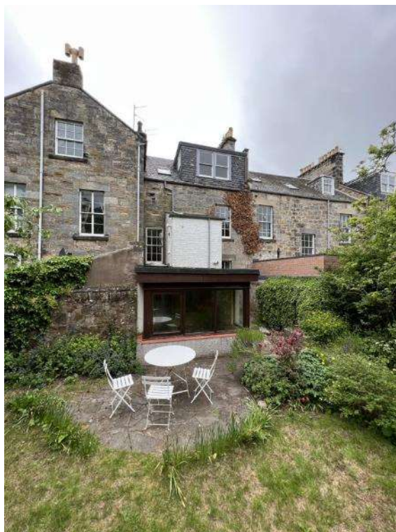
Plate 9: East elevation of 5 Queen's Gardens, looking west (RKA Architectural Design)
