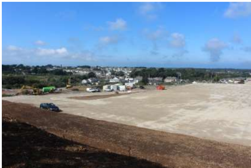
Figure 18: Trench 5 - car park and access road. View to north-west
