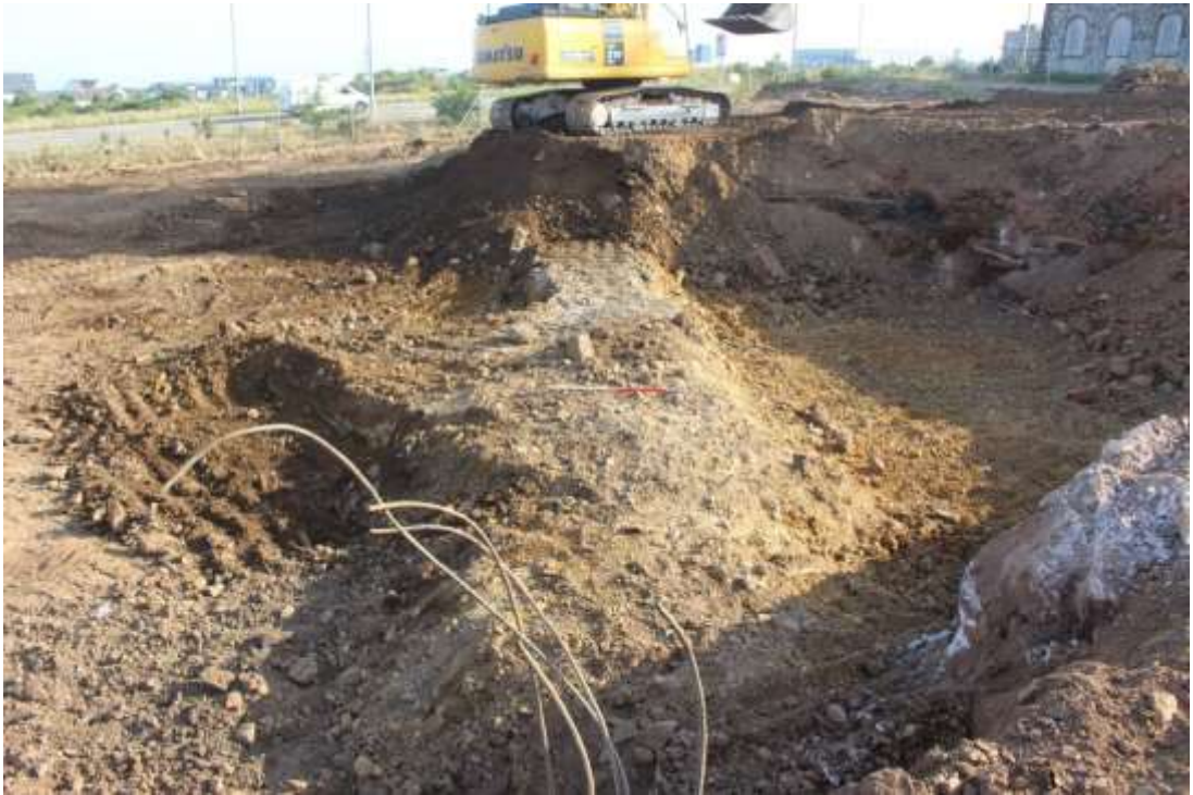
Figure 10: Trench 3, compacted stone railway footing 302. Scale at 1m. View to the north
