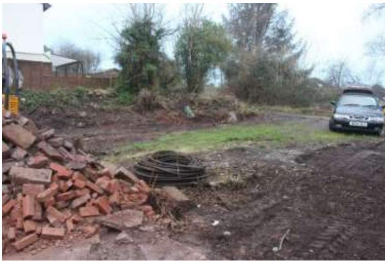
Plate 1: General view of site prior to works. View to the north-west.
