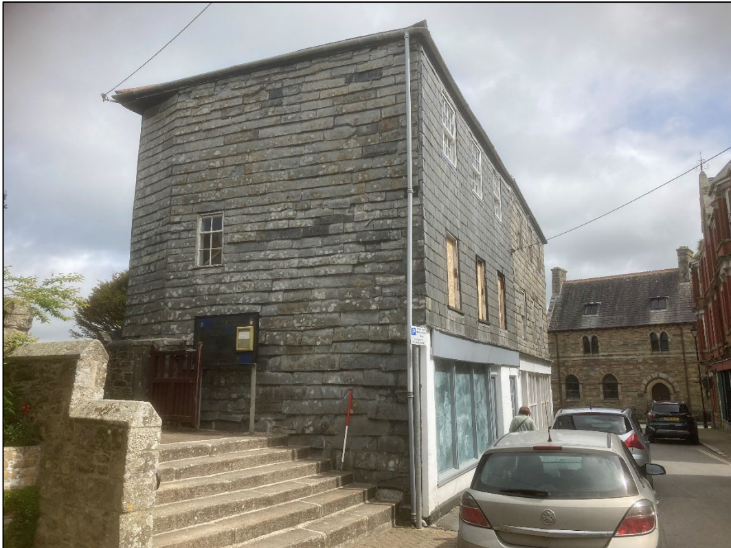
Figure 8: The buildings western elevation. View to the northeast
