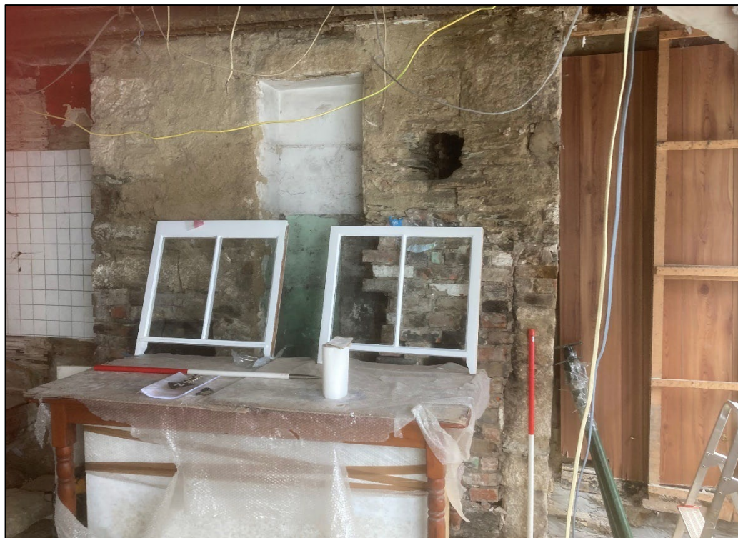
Figure 12: The eastern party wall. View to the east
