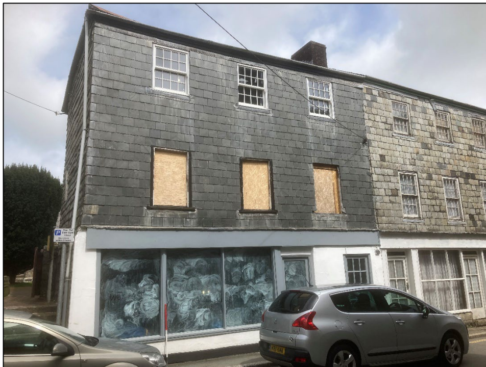
Figure 5: External view of the shop front, view to the north
