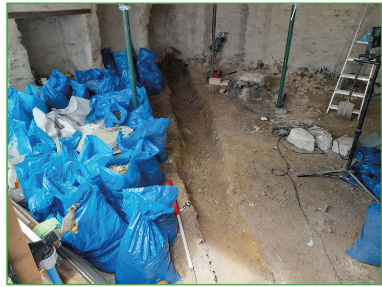
Post Excavation of Service Trench. Facing northwest (Scale at 1m)
