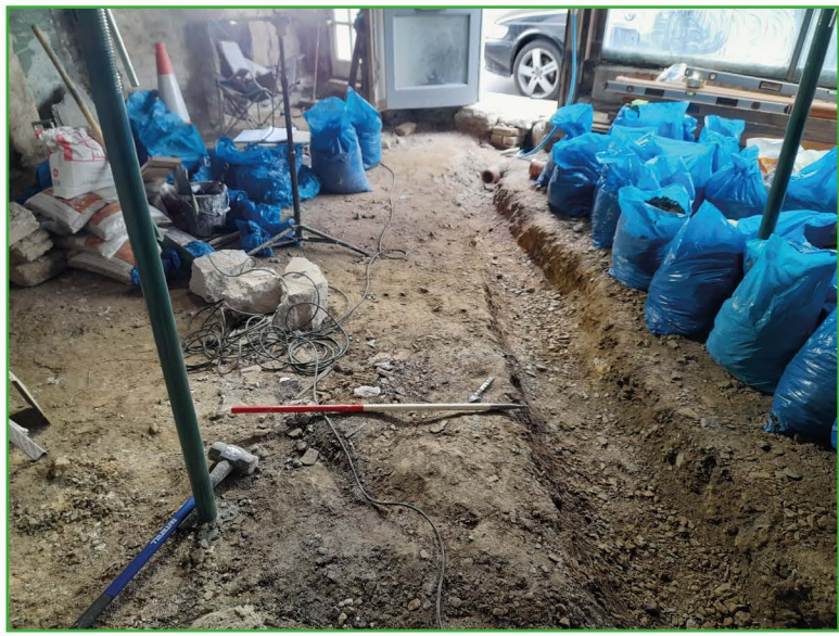
Post Excavation of Service Trench. Facing southeast (Scale at 1m)
