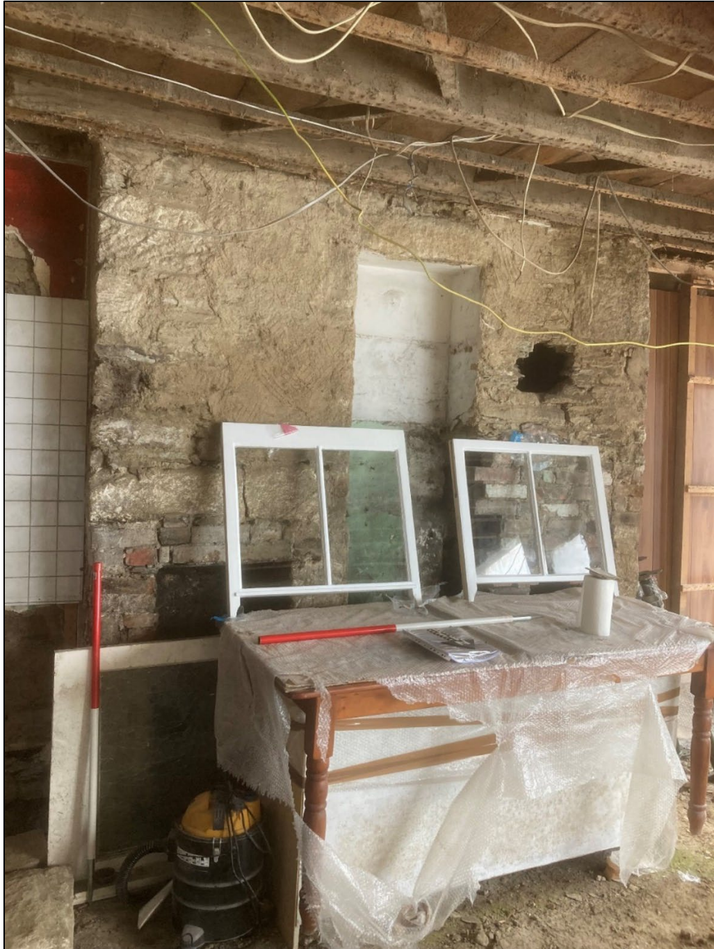
Figure 13: The eastern flue stacks. An iron strap lintel and repair work in red brick are present within the northern (left) stack. View to the east
