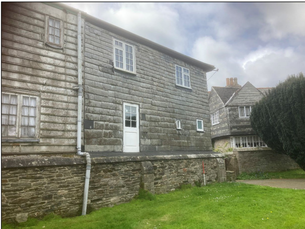
Figure 7: The buildings southern elevation facing the churchyard. View to the southwest
