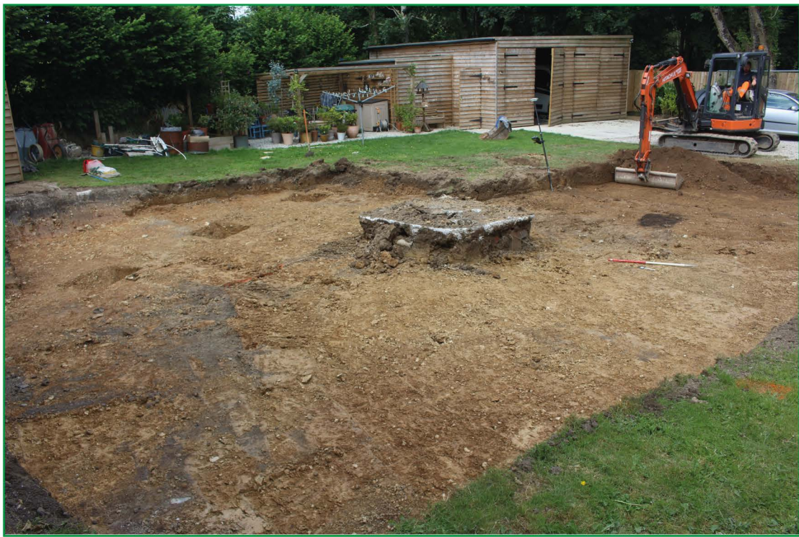
Scale at 1m. View to north-east
