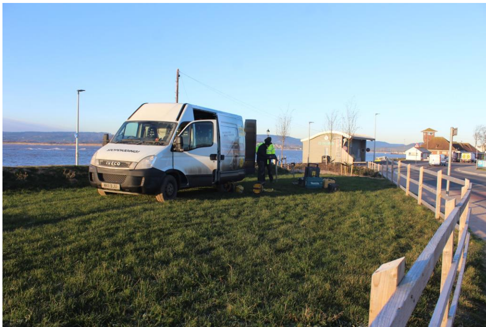
Plate 1: General view of site prior to works. View to the west.
