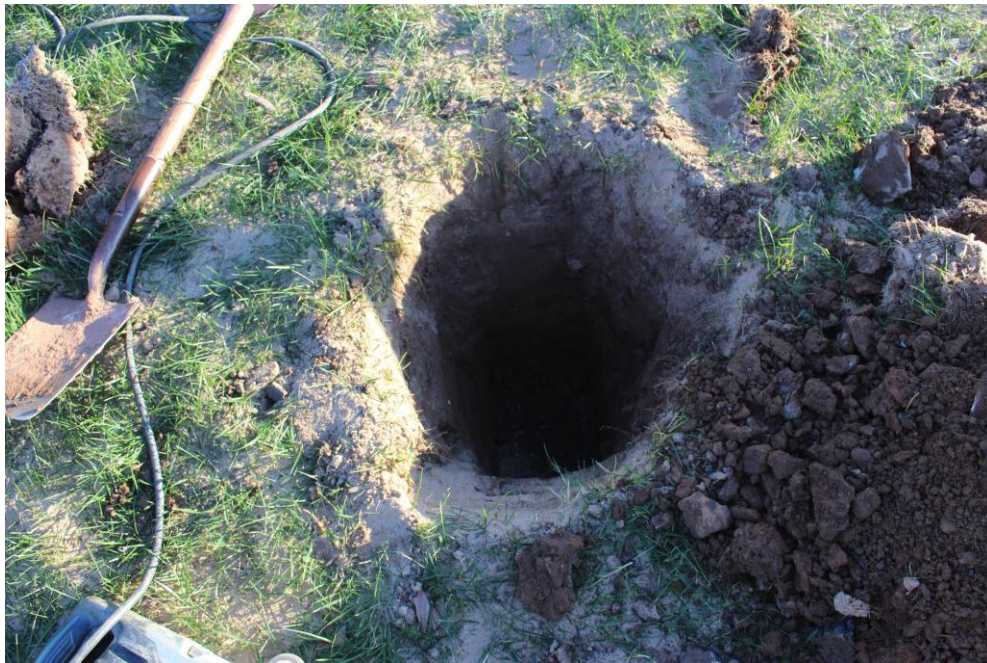
Plate 2: Screw test 4, hand dug hole through overlying deposits, to top of tarmac layer. View to the north-east.
