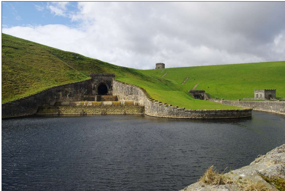
Plate 3: general arrangement showing the overflow tunnel (left) and outlet tunnel (right) with draw-off tower above
