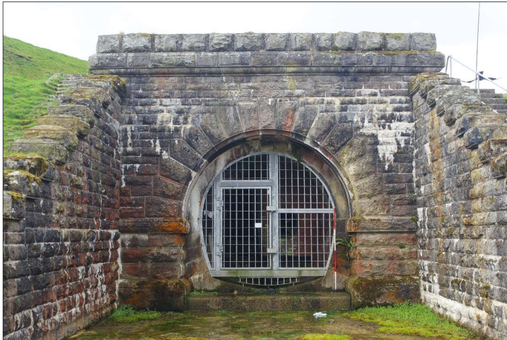
Plate 4: the portal facing west
