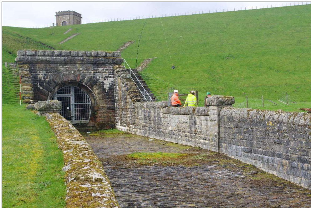
Plate 5: the portal, side walls and channel
