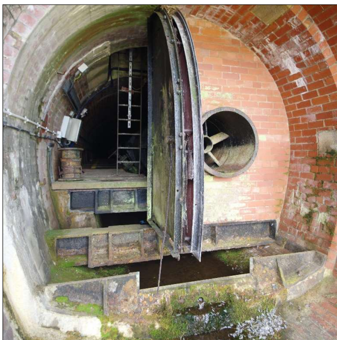
Plate 7: tunnel interior facing west
