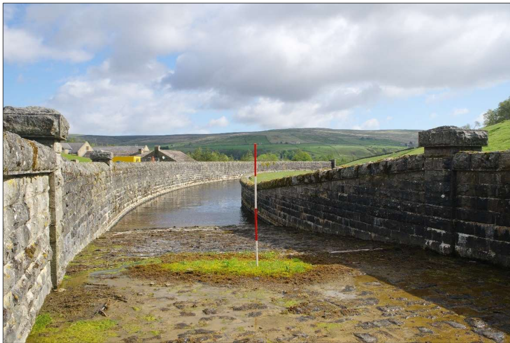
Plate 6: tailbay channel facing north-east
