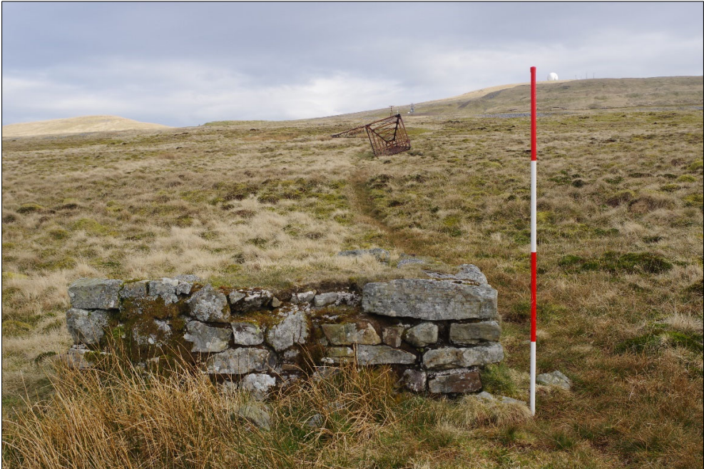
Plate 12: Pylon 4, base facing north with displaced pylon to the north
