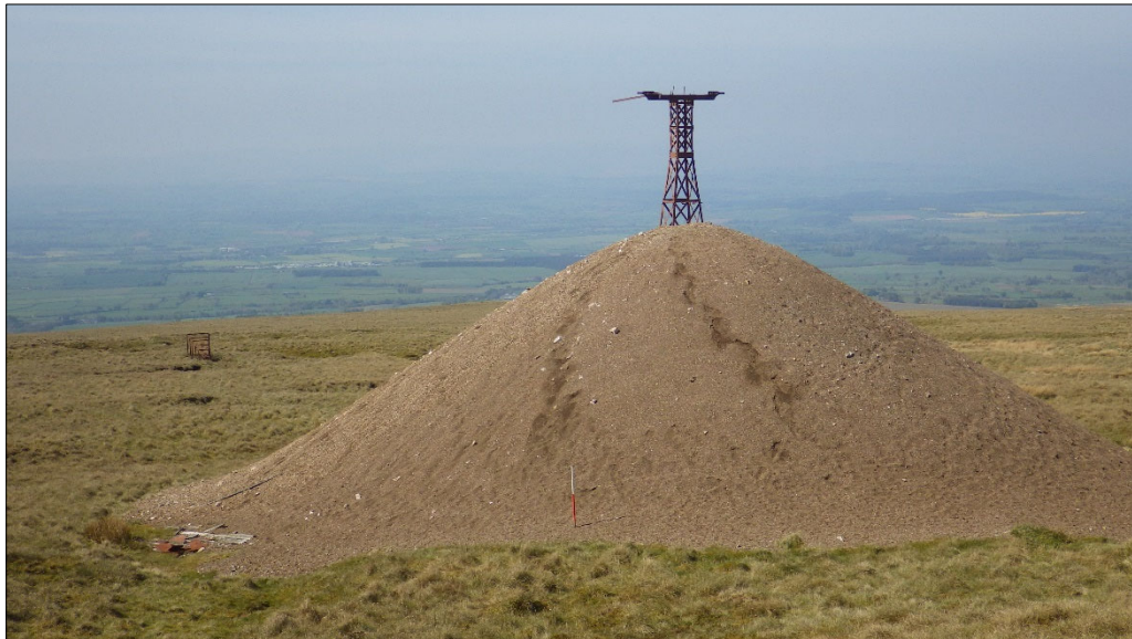
Plate 10: Pylon 1, facing south, photographed in 2019; Pylon 2 is visible on its side, left of the photograph
