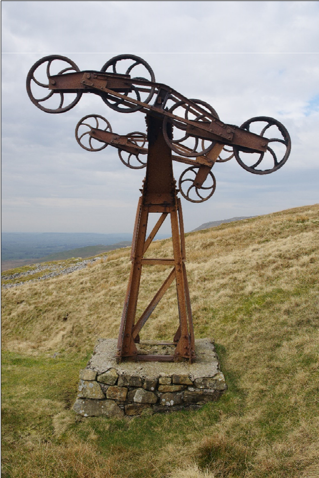
Plate 13: Pylon 12, facing west
