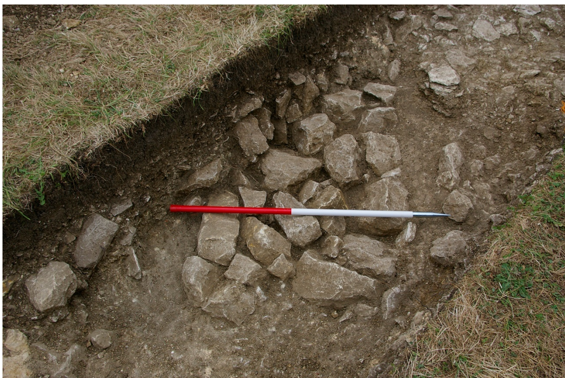
Figure 24 Possible wall footings (6008) (from SE)
