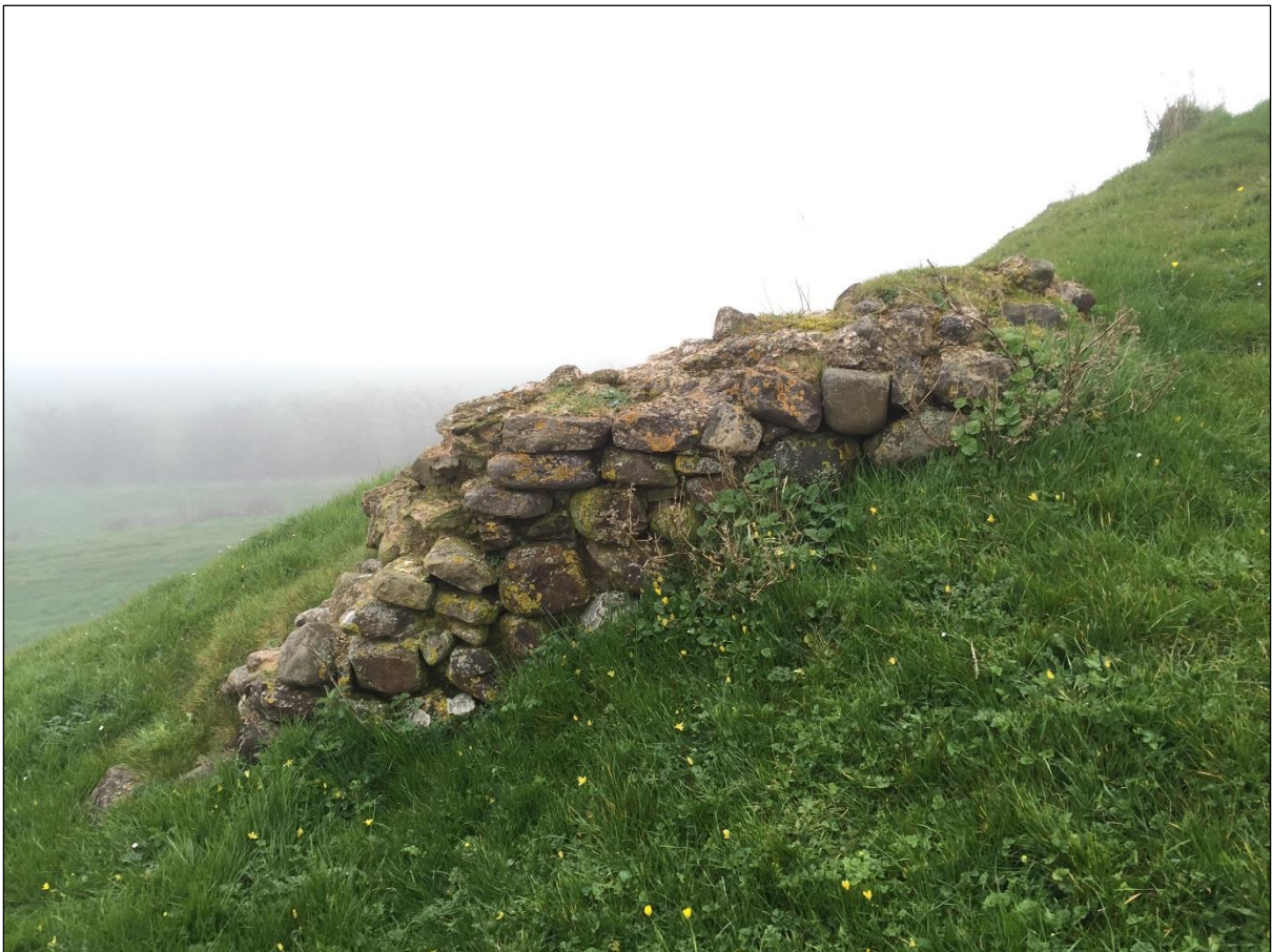
Figure 2: Skipsea Castle: section of cobble walling.
