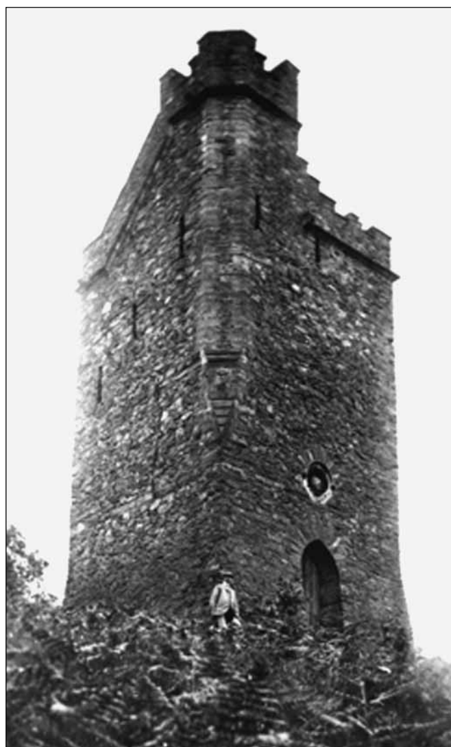
The prominent granite memorial tower erected at Cademan Wood near Temple Hill, Charnwood, in memory of Everard Aloysius Lisle Phillipps. Now demolished. (Reproduced by permission of Whitwick Historical Group.)
