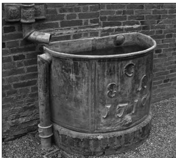
Lead water cistern on the south side of Belgrave Hall bearing the initials C E A and the date 1710.
