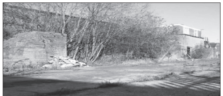
A rather forlorn looking picture of the 'new' reinforced building on Abbey Lane from 2010. (Photograph online on 28 Days Later Forum, unable to trace original source.)
