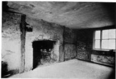
B. Fireplace in West Wall of Upper Storey, No. 2 Bosworth House.
