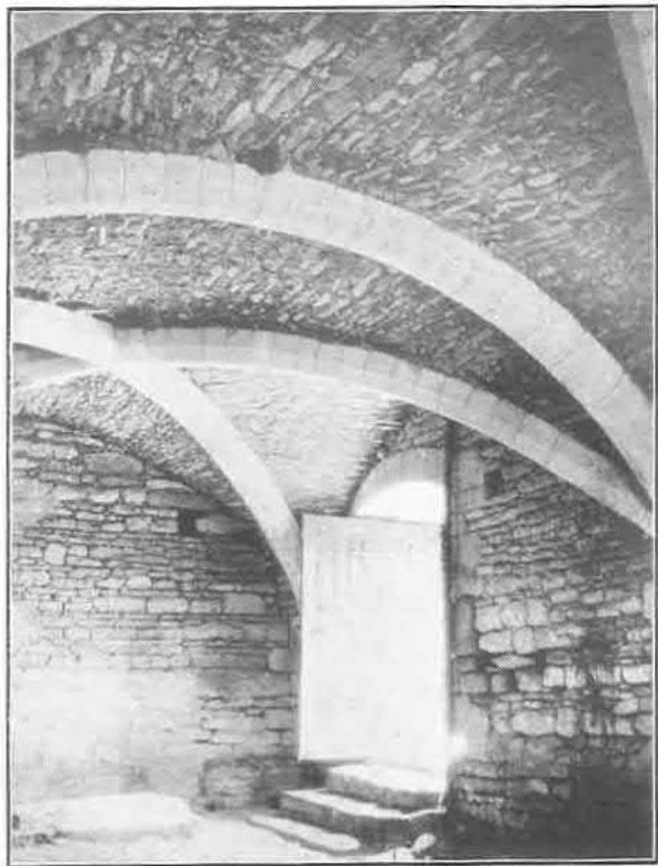
Ground Floor—Boothby Pagnell Vaulting under Hall on Upper Floor, C. 1180
