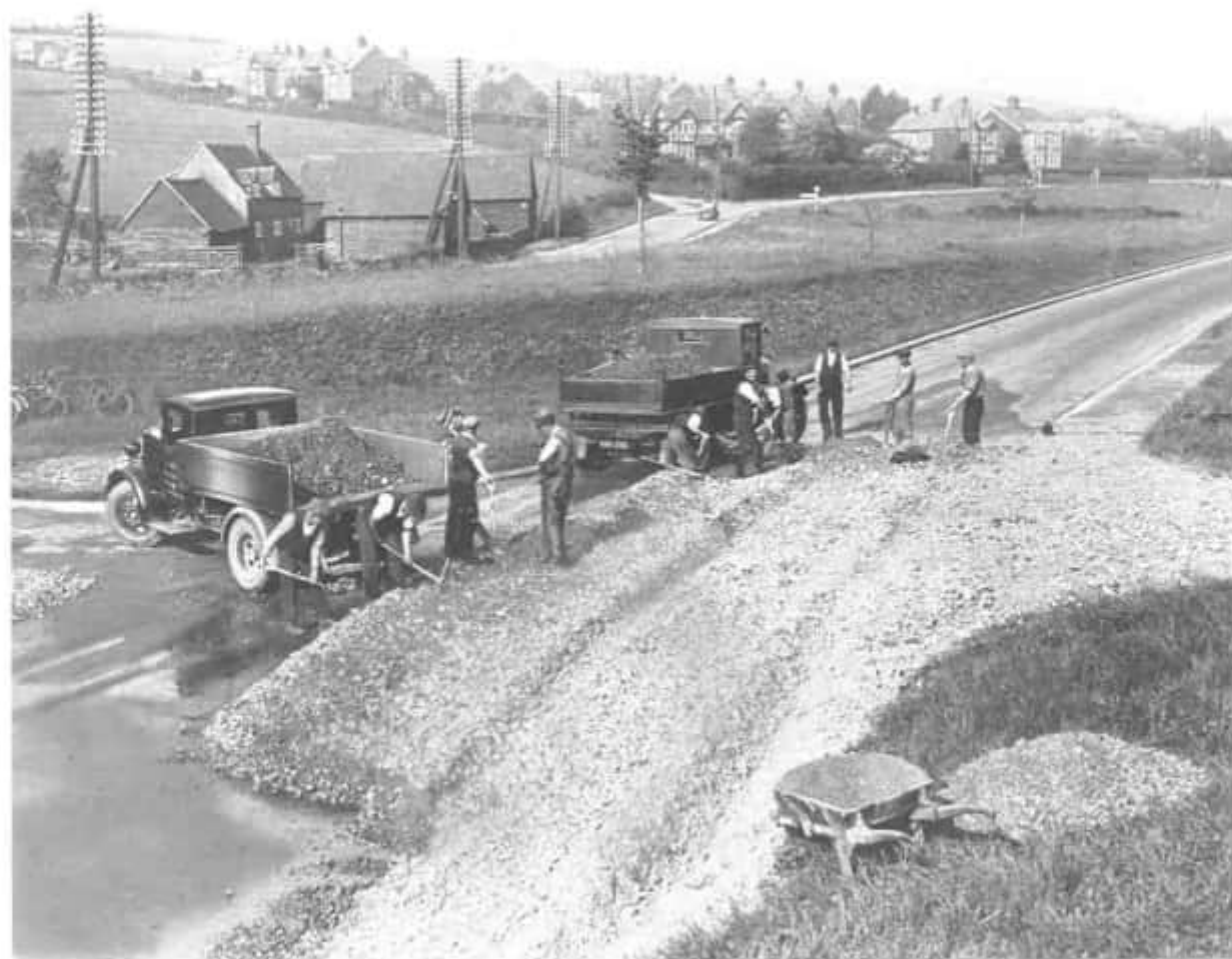
Diddington: de'ta-fan of gravel in course of removal from Oxford after cloud-burst on 17 May, 1936
