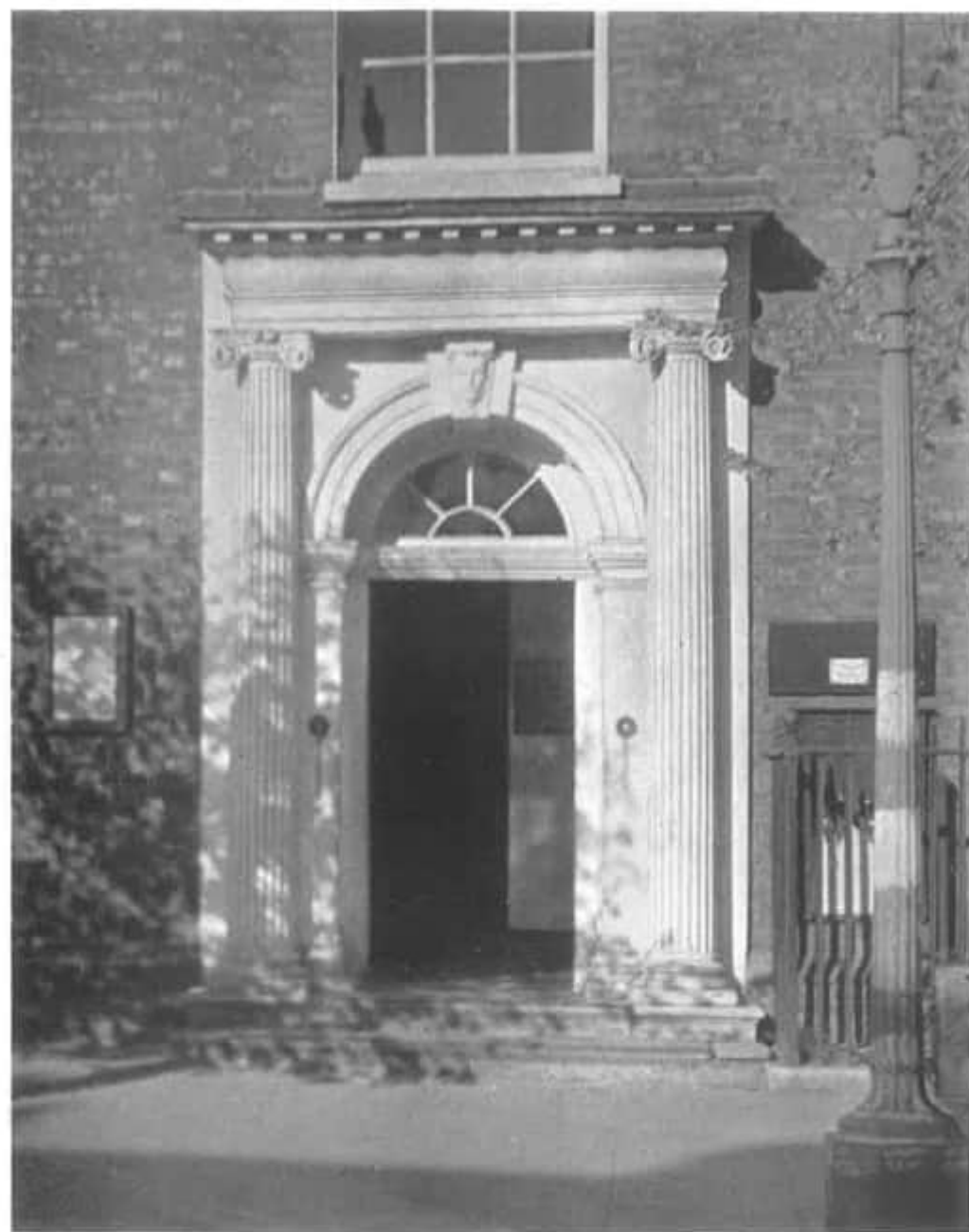
PLATE 2. MARLOW POST OFFICE: THE DOORWAY
