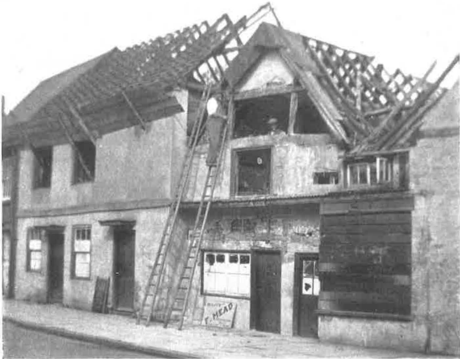
PLATE 2b. CHALFONT ST. PETER, HIGH STREET. The house described in this article in course of demolition. The text, rose and thistle have just been removed from the panels above the main tie-beam in the gable
