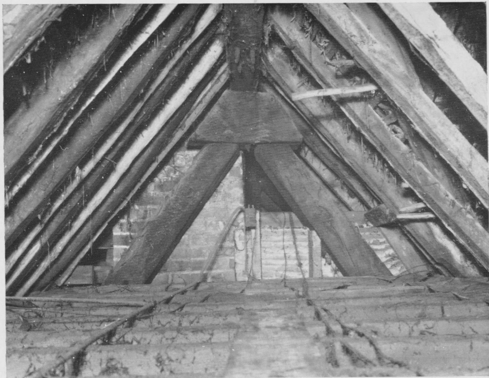
PLATE Xa. CHALFONT ST. PETER. Hill Farm. Apex of cruck truss.
