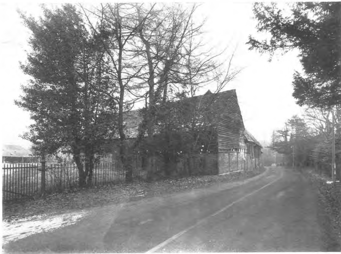
PLATE VI. Hitcham Barn from the South West
