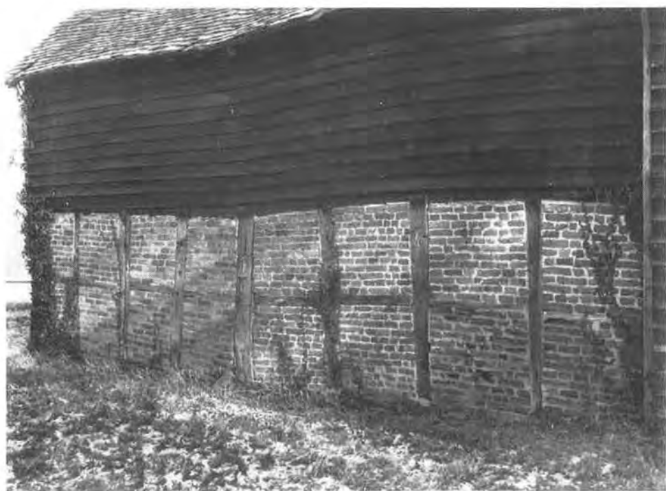
PLATE VIII (b). Detail of West Elevation. Brick filling built after settlement of foundations.
