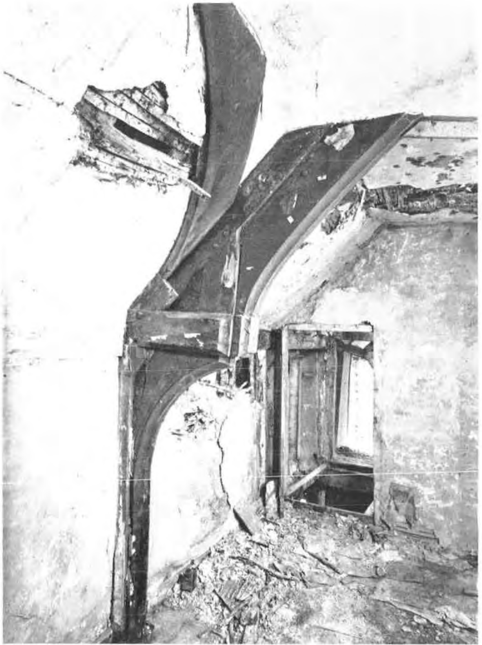
PLATE II. Hammer-beam joint (phase 2).
