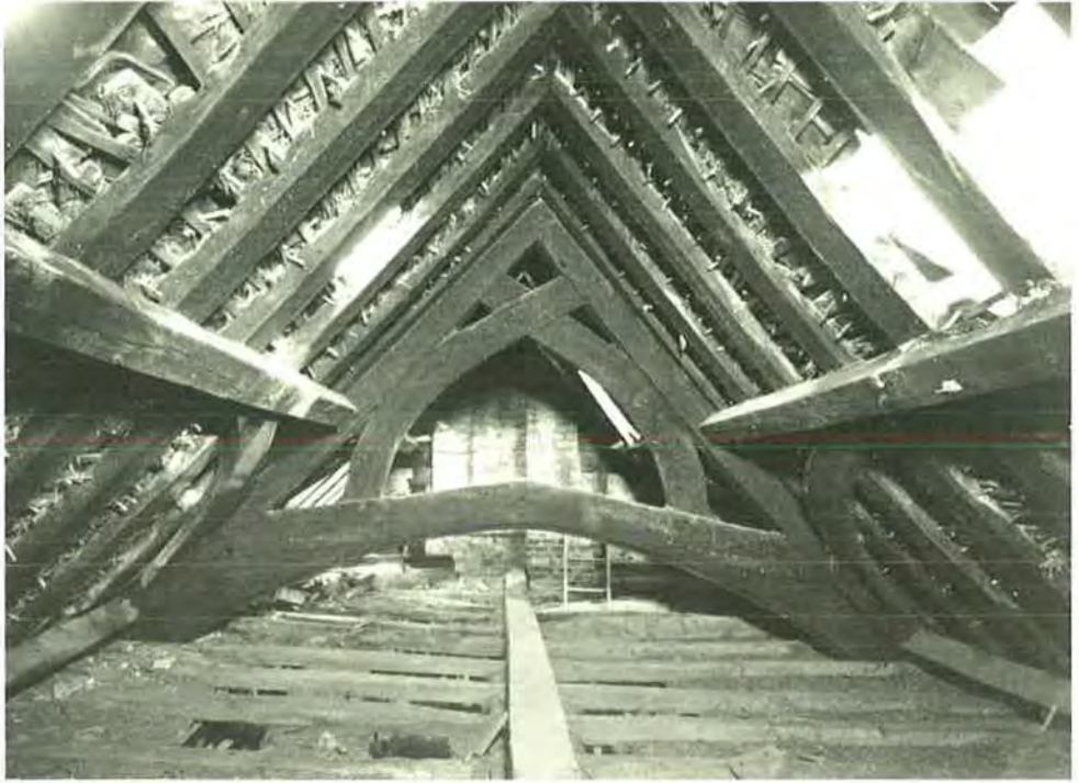
PLATE IV (a). Bracing above the collar on the hammer-beam truss.
