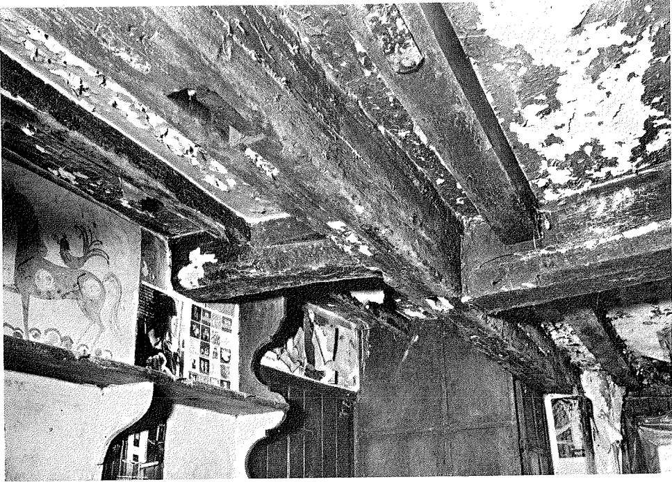
Plate Va. Original end wall beam with mortises. Ground floor N room.
