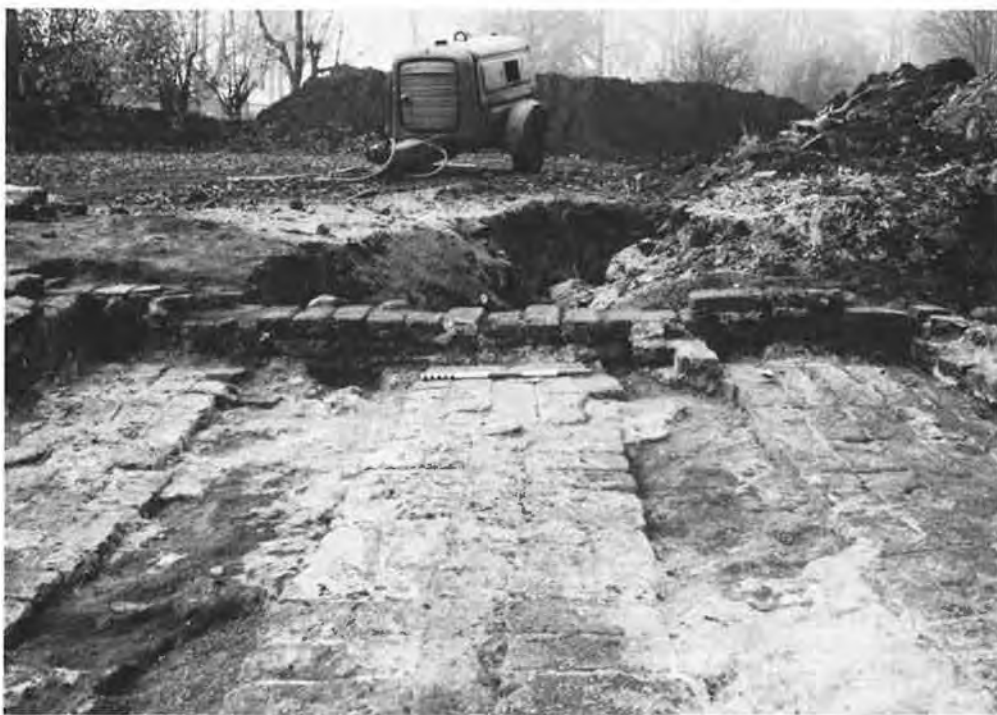
Plate XXI. Detail of west wall of kiln 2, with wall stub 43 and both wall channels.
