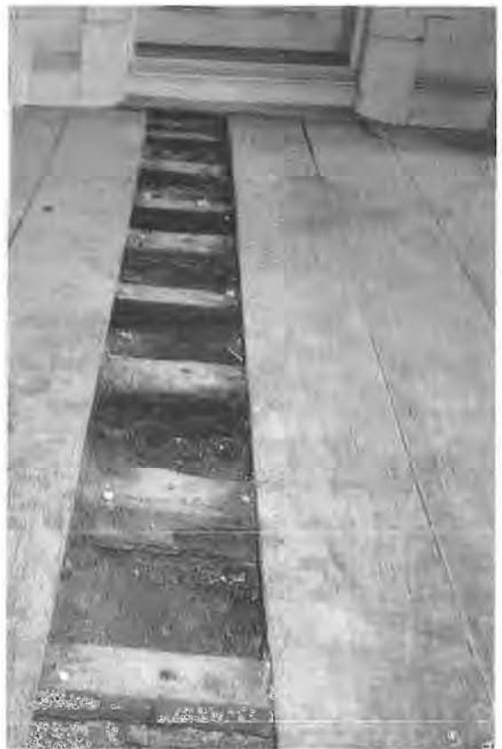
Plate IV. Rafters re-used as floor joists, Grinnell Room, showing peg holes for sprocket.
