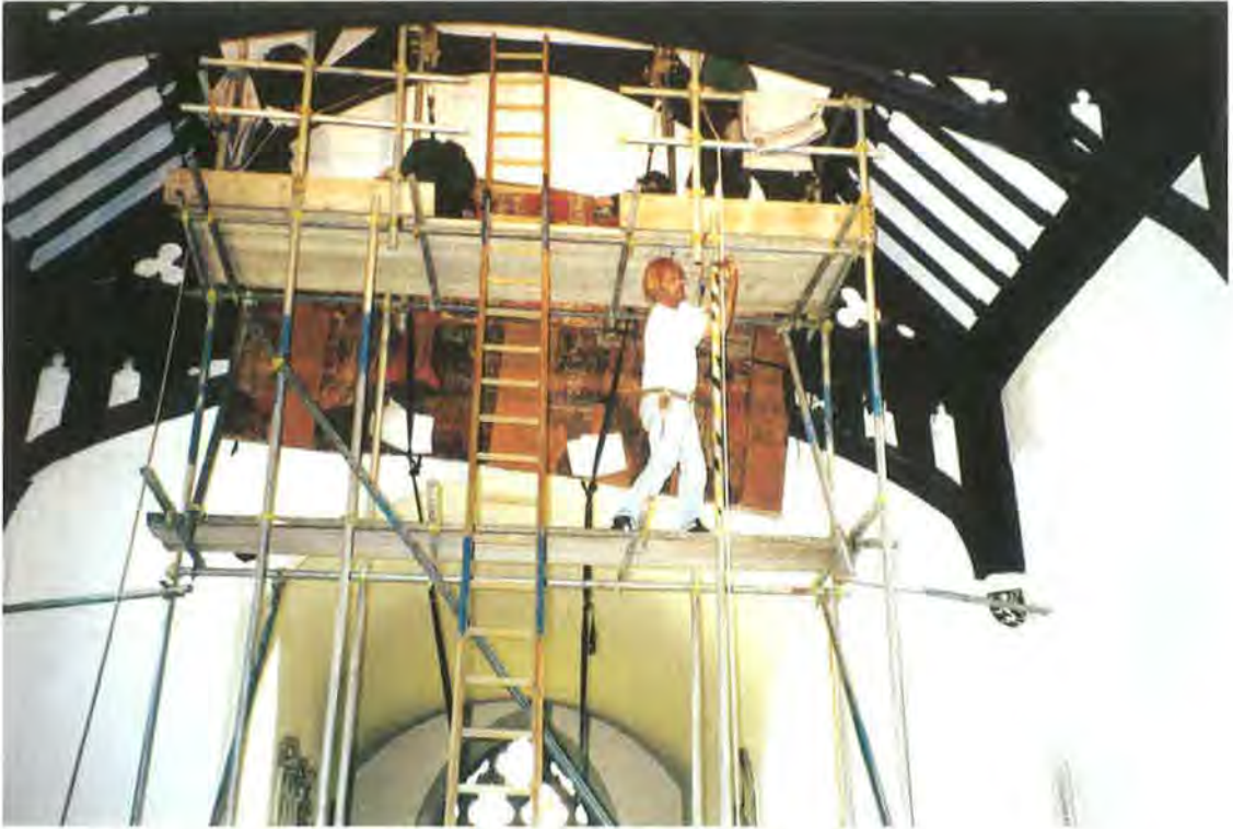
FIGURE 10 The Doom being taken down from above the chancel arch prior to its recent examination and conservation. To the right can be seen the Rood loft entrance set between the corbel supporting the tie beam and a clerestory window. (Photo by John Wood).
