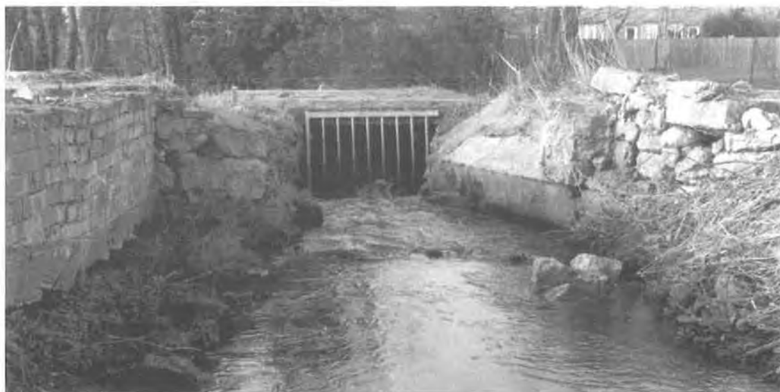
PLATE 2 The mill stream running north-west towards the former mill complex.
