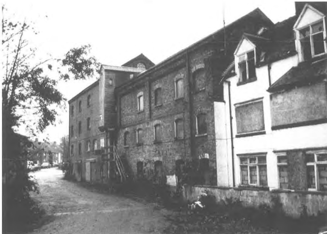
PLATE 1 The Oxford Road mill as photographed in 1991, looking north east (copyright Mike Farley).
