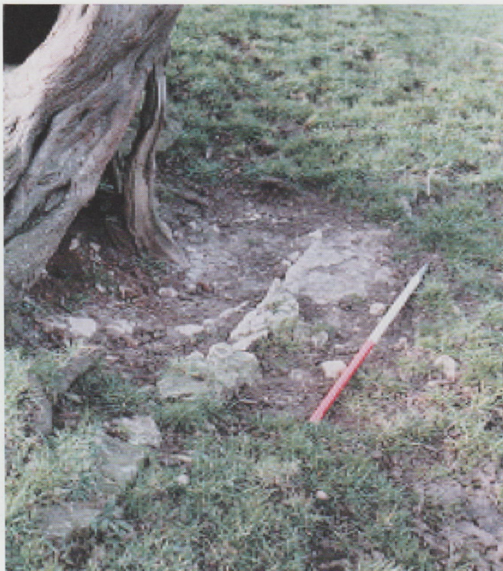
PLATE 5 Detail of the exposed wall facing on the crest of the bank flanking the western side of the lower garden.
