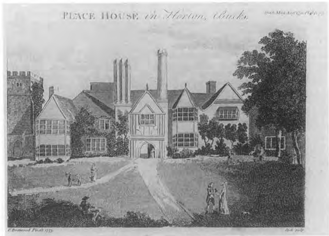
FIGURE 1 Upper: Place House, Horton circa 1705. Reproduced courtesy the Bodleian Library (Ms. Top. Bucks, c.1. f.54 facing.) Lower: Place House, Horton in 1773. Print in BAS collections ( BAS 4/56)
