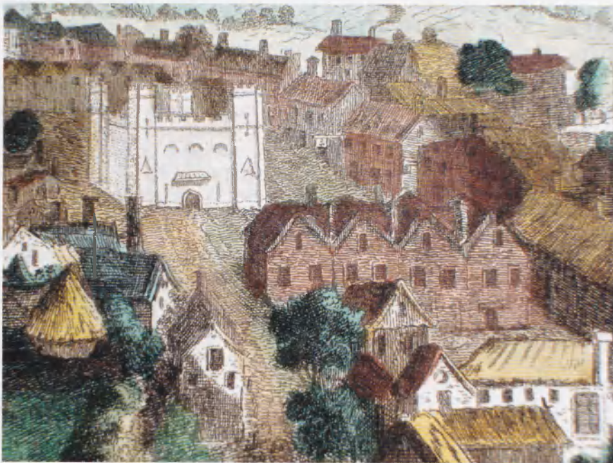
FIGURE 3 Upper: Bickham's views of Buckingham 1753. Lower: Detail of The Red Buildings opposite the Gaol.
