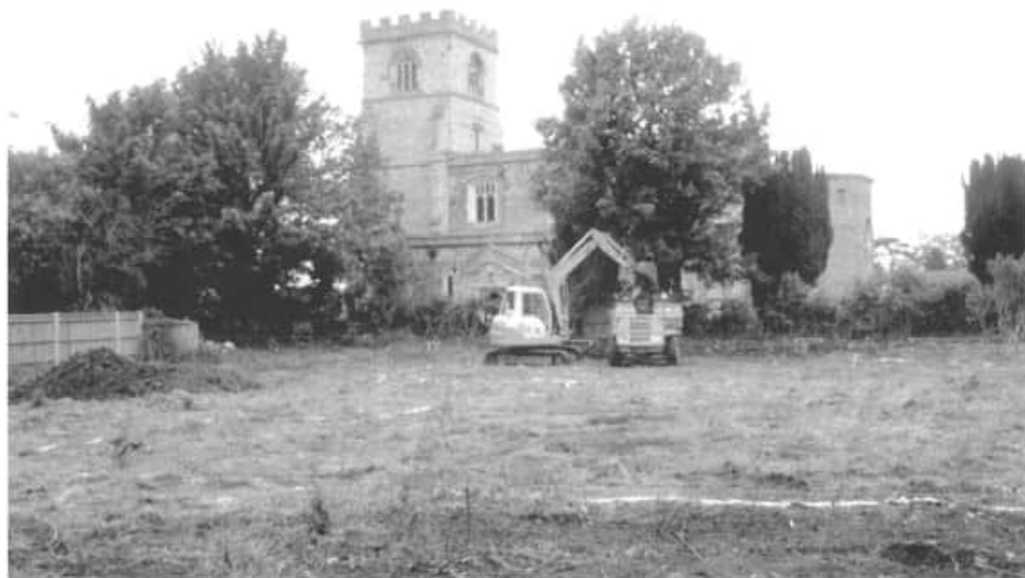
FIGURE 4 The cemetery area at the beginning of soil stripping with mechanical excavator and dumper
