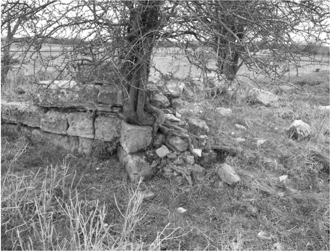
PLATE St Peter's Church, Quarrendon: ruins at risk from tree roots (the bush has since been removed as part of the conservation work)
