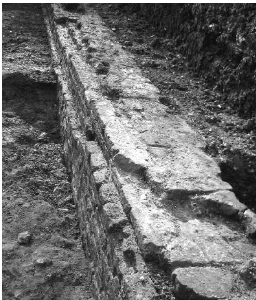
FIGURE 8 A View along the post-medieval wall uncovered in Trench 3. Note the moulded brick special, probably part of a mullion window, incorporated into this structure. The surface of medieval pit can be seen protruding from under the wall and marked by the cluster of animal bones protruding from the surface.
