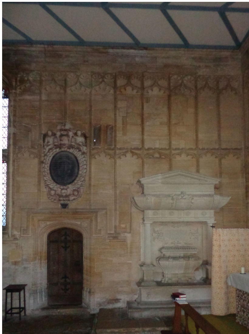
FIGURE 5 The north wall of the north chapel, showing the door to the closet and vestry block and the windows of the closet, partly blocked by the later monument above the door. (photo: Vicki Harding)
