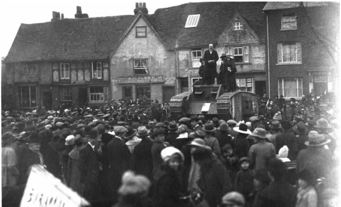
FIGURE 2 The Aylesbury Presentation Tank being installed in Kingsbury Square, 24 March 1920 (photo: Centre for Bucks Studies)
