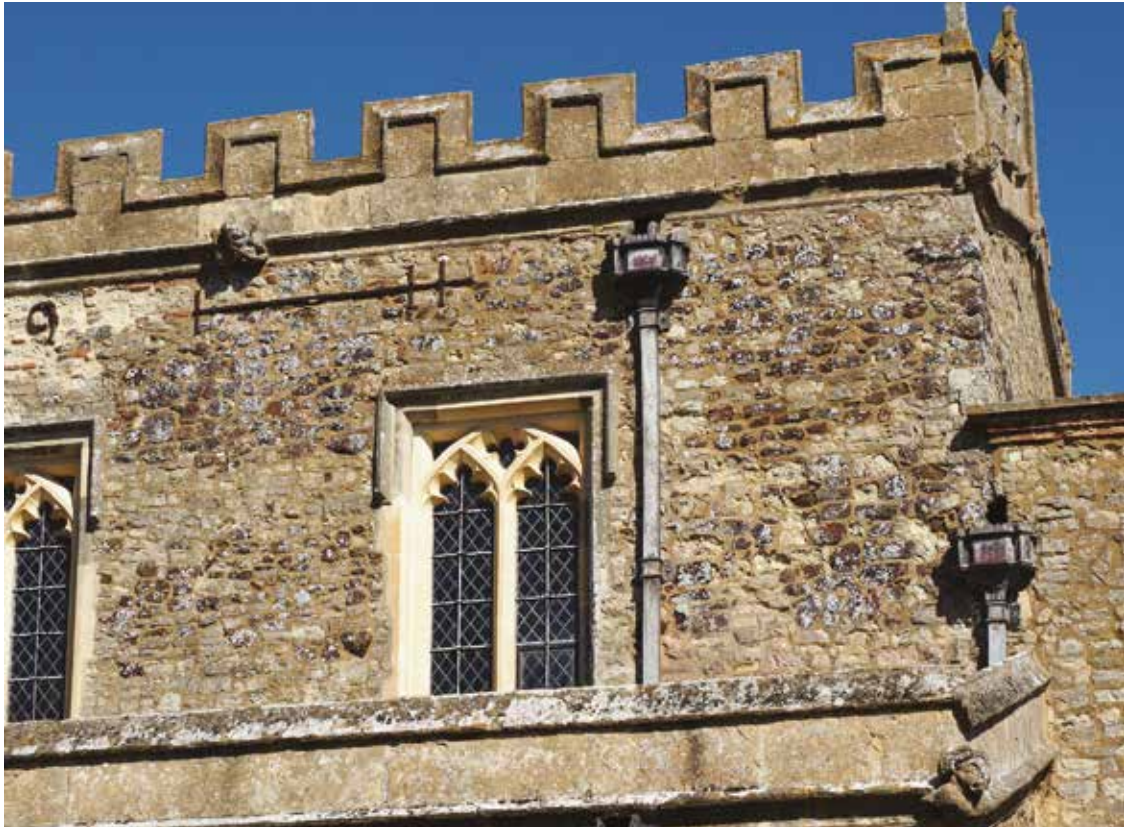
FIGURE 10 SE angle of nave clerestory with apse butt-jointed against it
