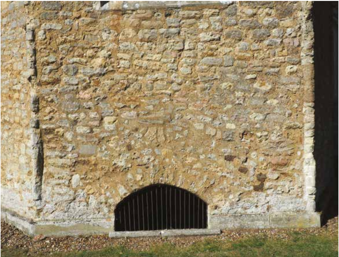
FIGURE 3 Irregularly pitched masonry around window in E bay of the apse
