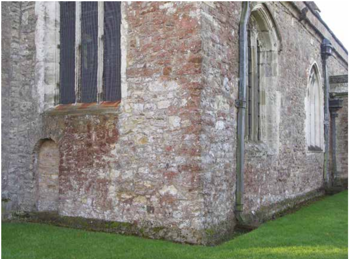
FIGURE 6 E end of N aisle, incorporating masonry of former NE porticus
