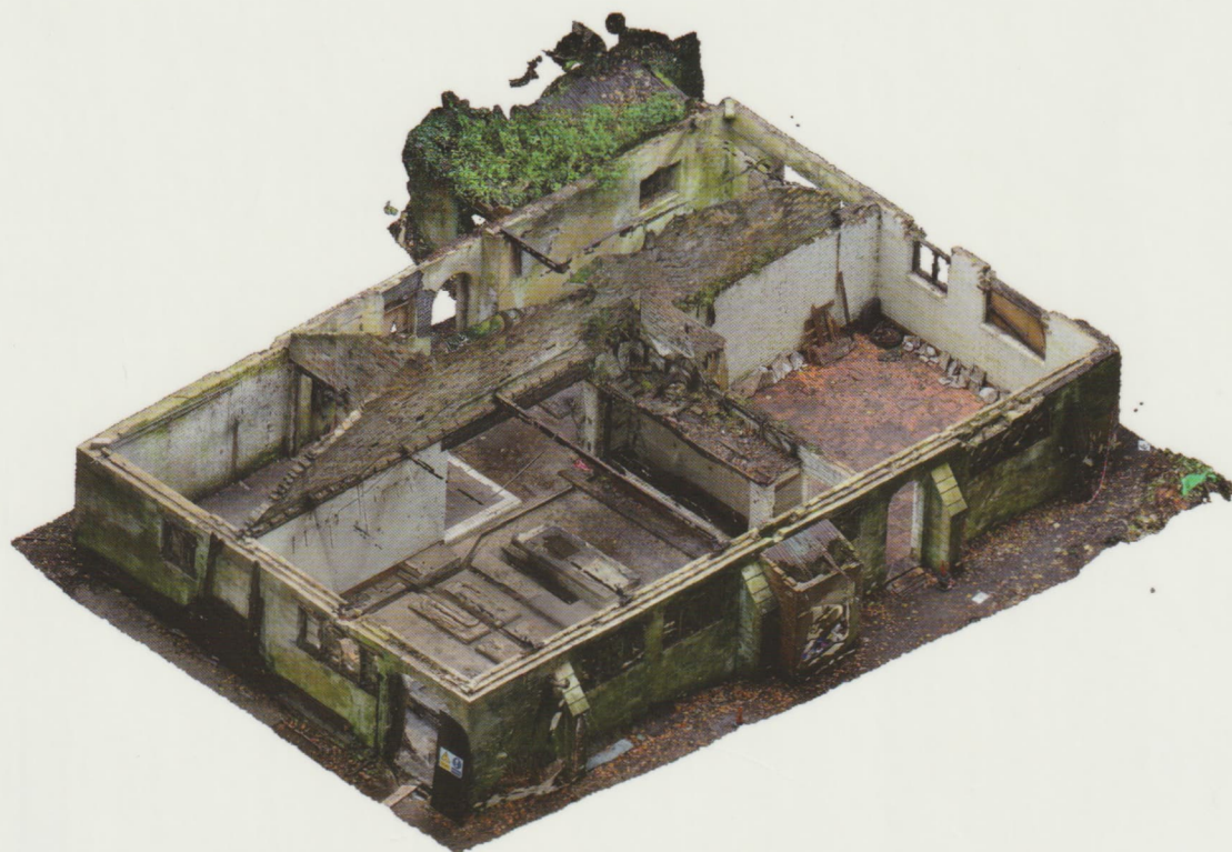
Generator house, Cliveden: bird's eye photogrammetric view looking north
