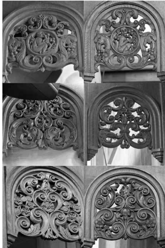
FIGURE 34 Openwork infillings of the screen side arches (north screens at top, south-east screen at bottom)
