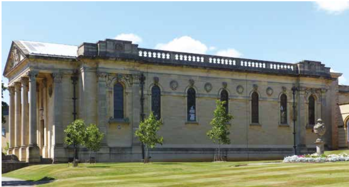
FIGURE 1 View from the south-east in July 2017
