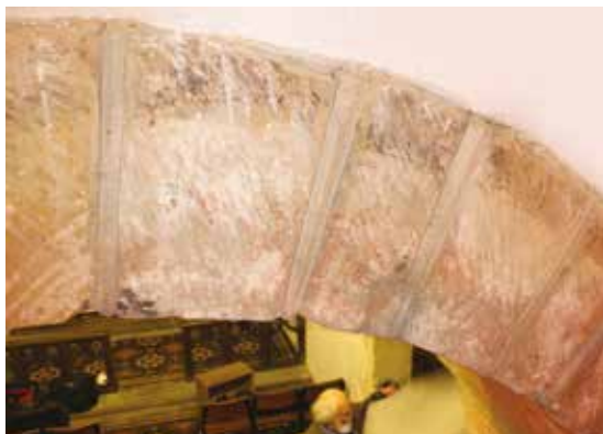
FIGURE 12 Detail of S side of arch, showing distinctive dark outer band of original scheme, with a fine white line along its inside edge. Red on the inner areas belongs to a later painting scheme (EH)
