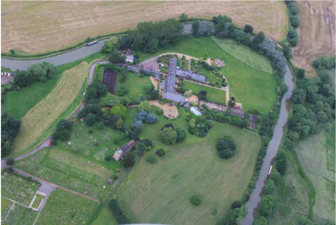
FIGURE 1 Aerial photograph of the site of the church and manor, bounded by loop of the Grand Union Canal (Mike Farley)
