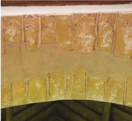
FIGURE 6 The soffit of the chancel arch (RG)
