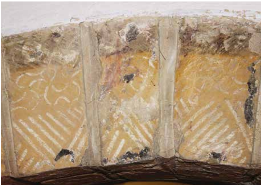
FIGURE 11 Detail of original polychromy on voussoirs 7, 8 & 9 in three distinct bands, with small patches of later overpainting in red and black (EH)
