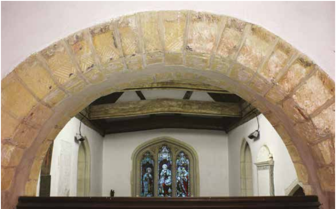
FIGURE 10 Overall view of surviving polychromy on central section of the arch (EH)
