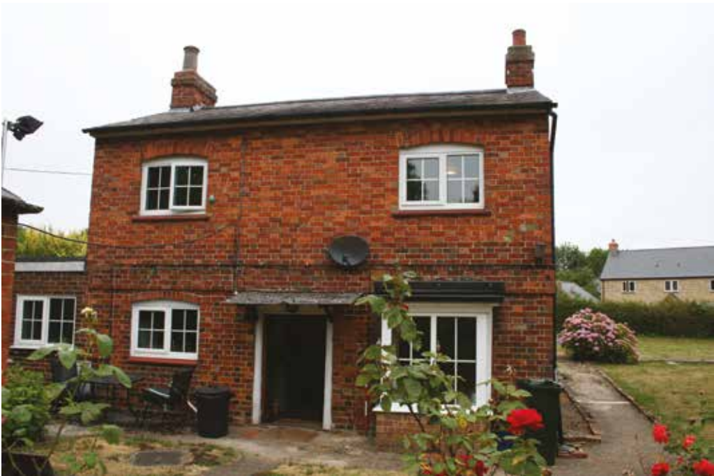
FIGURE 14 The lock-keeper's cottage, south elevation, 2018
