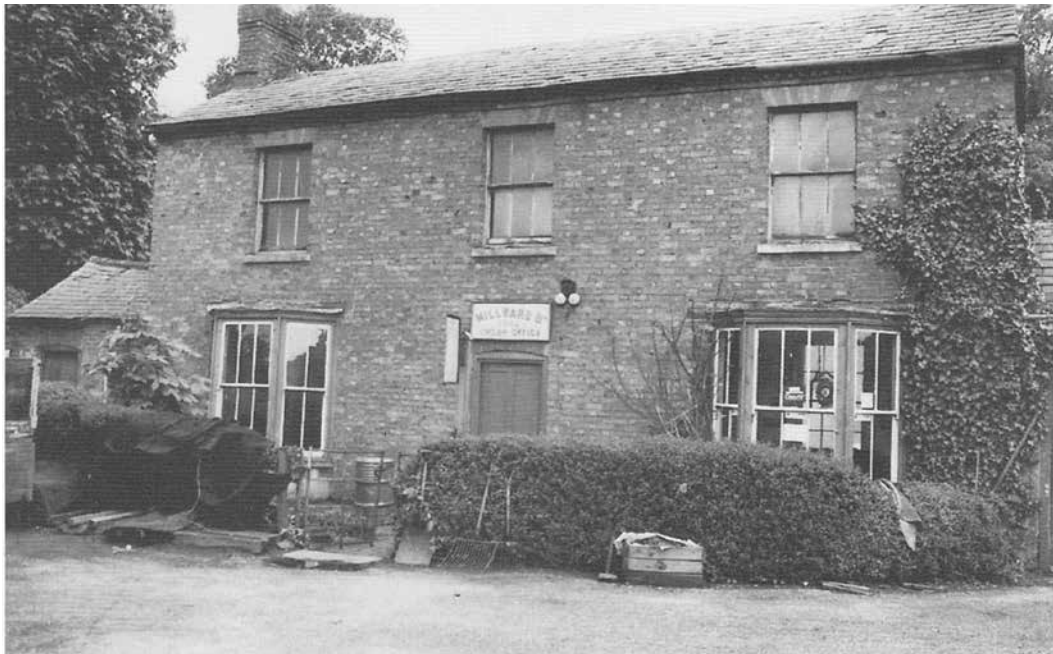
FIGURE 9 The wharfinger's house at Hives' Wharf, Newport Pagnell
