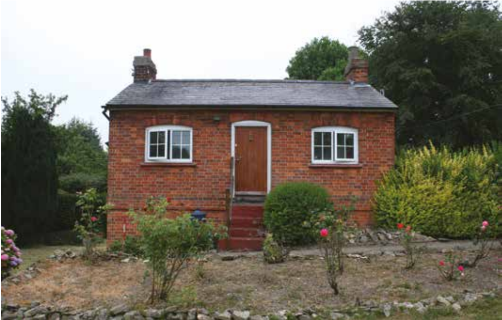
FIGURE 13 The lock-keeper's cottage, north elevation, 2018
