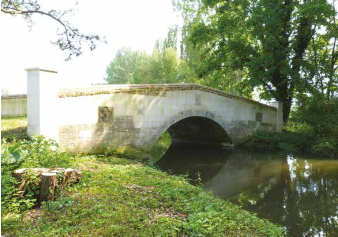
FIGURE 4 Nether Winchendon Manor: Thomas Harris's fine bridge, c.1802 (S Tricks)
