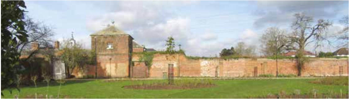
FIGURE 1 Baylis Park, Slough: early to mid-18th century garden pavilions and walls. It is now a public park (S Rutherford)
