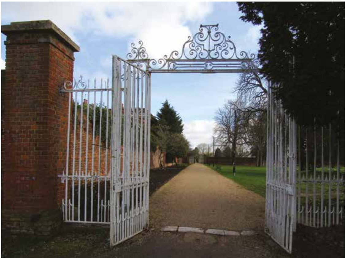
FIGURE 2 Baylis Park, Slough: early to mid-18th century iron garden gateways and walls (S Rutherford)
