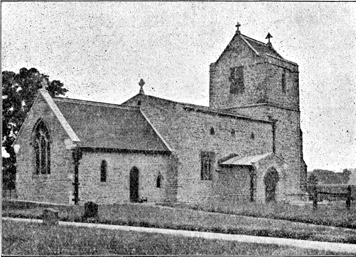
BRADWELL CHURCH, AFTER REPARATION. N.E. VIEW.
