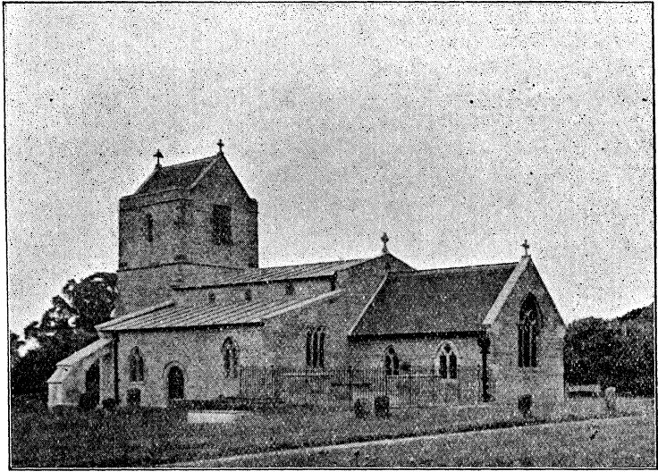
BRADWELL CHURCH, AFTER REPARATION. S.E. VIEW.
