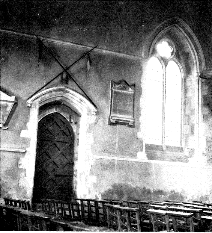
ALL SAINTS CHURCH, HIGH WYCOMBE. NORTH DOOR AND NORTH AISLE WINDOW.
