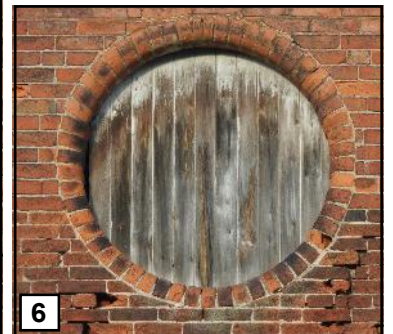
Plate 5: The sawtooth brickwork beneath the eaves. Plate 6: The circular pitching hole in the south elevation, Bay 1, viewed looking north.
