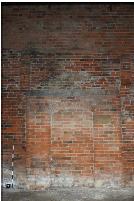
Plate 14: The winnowing doorway viewed looking north.
