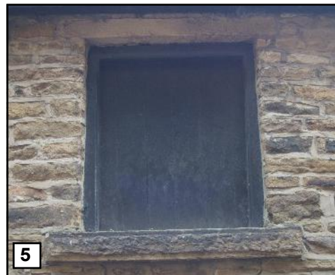
Plate 4: The blocked winnowing door in the north elevation, viewed looking south.
