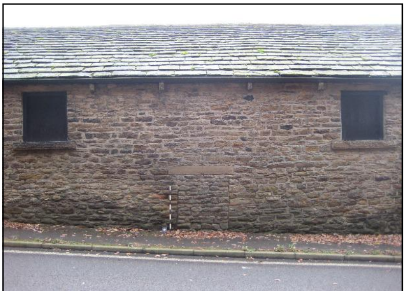
Plate 3: The north elevation, viewed looking south.
