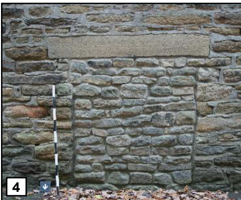
Plate 4: The blocked winnowing door in the north elevation, viewed looking south.
