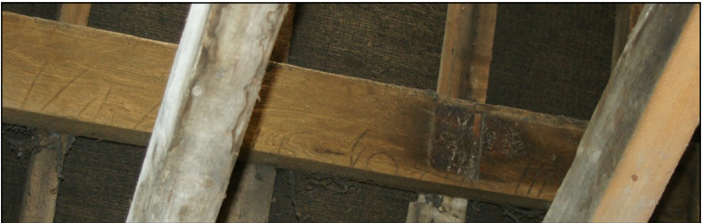
Plate 14: Baltic timber consignment marks on the northern purlin in the western half of the East Section.
