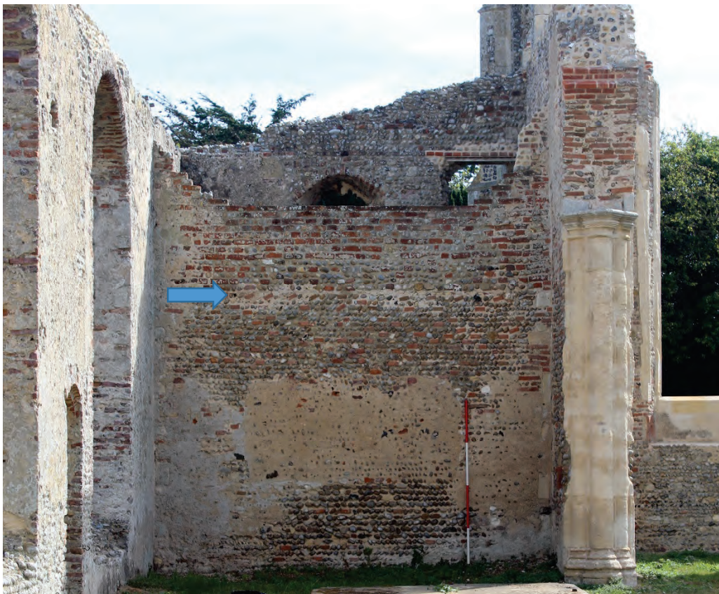
Plate 22. East wall of the chapel in the north aisle inserted after the exterior wall of the north aisle was built. The top half of the wall was later taken down to first level (arrowed) and rebuilt sometime in the post medieval period. In 1678 Edward Barker was paid five shilling plus a further nine shilling for materials and expenses 'for skrewing up the wall in the north aisle' – the brick size for the upper part of the wall would fit this date but a 'skrew' is a coping stone.
