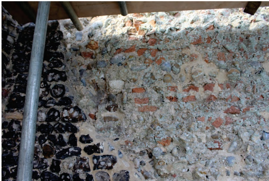
Plate 7. Brick rubble core beneath the dressed black flint of the chancel south wall
