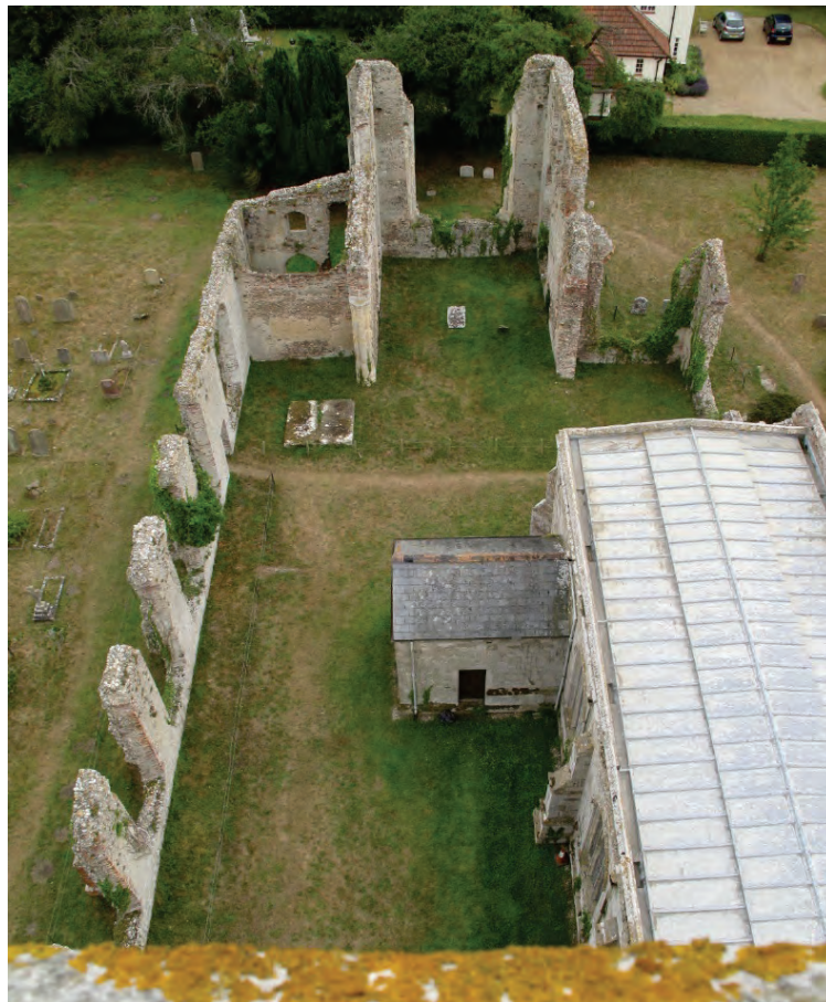
Plate 1. Ruins of the 15th century church of St. Andrew, Walberswick looking east from the tower. The roofed building on the right is the present parish church constructed in 1696 within the south aisle from stone salvaged from the earlier church. (Photo supplied by Nicholas Jacob Architects)
