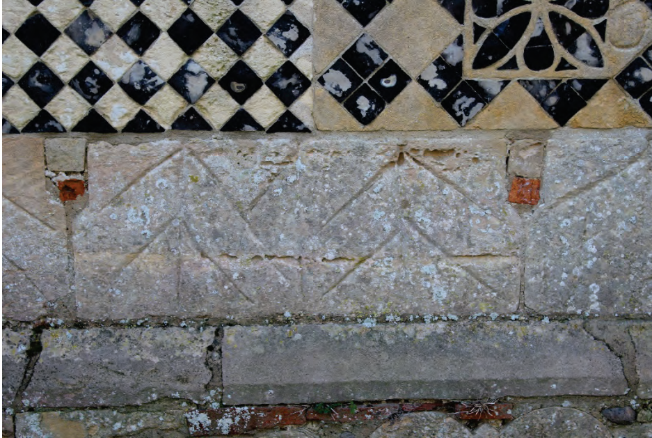
Plate 23 (?) Superstitious marks scratched on the stones below the east window of the 17th church
