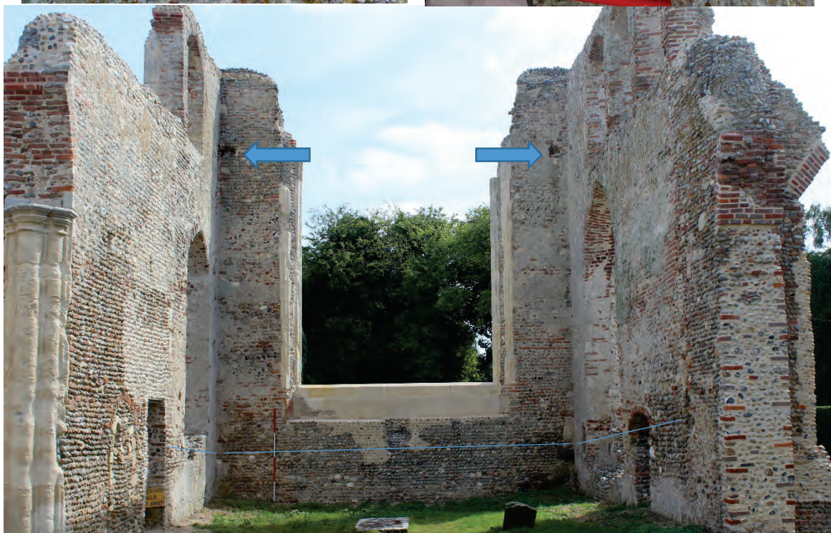
Plate 10. The Chancel looking east (bottom). The picture top left shows the line of the wall post, evidenced by the limit of the plaster (M). The sockets, which were at the mid-point (N) and base of the post (P), are for an attachment point and corbel respectively. The picture top right shows the line of the corner post (K) as a break in the plaster, large ragged holes at the base of the corner posts are probably for corbels (I and J). The letters used to annotate the photographs correspond with those used on the drawing in figure 3. The corbels at the base of corner post are highlighted in the lower picture and a change in a phase of built marked with a blue line.
