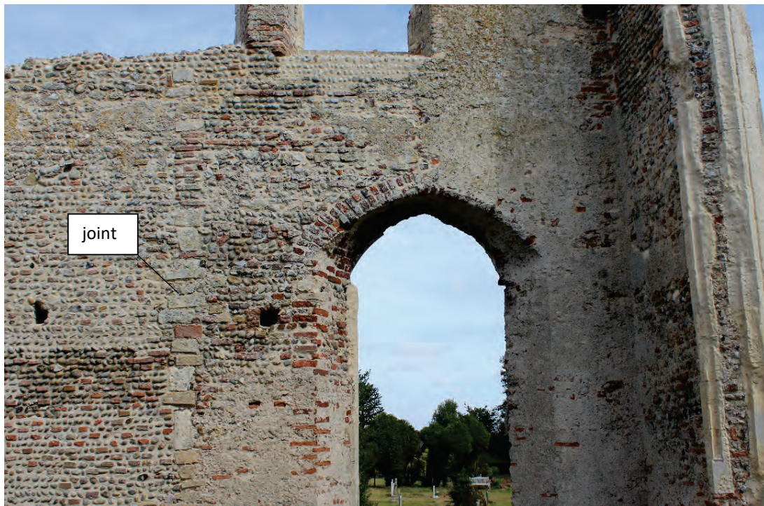
Plate 17. Joint between the chancel (right) and Sacristy walls stitched together with limestone blocks
