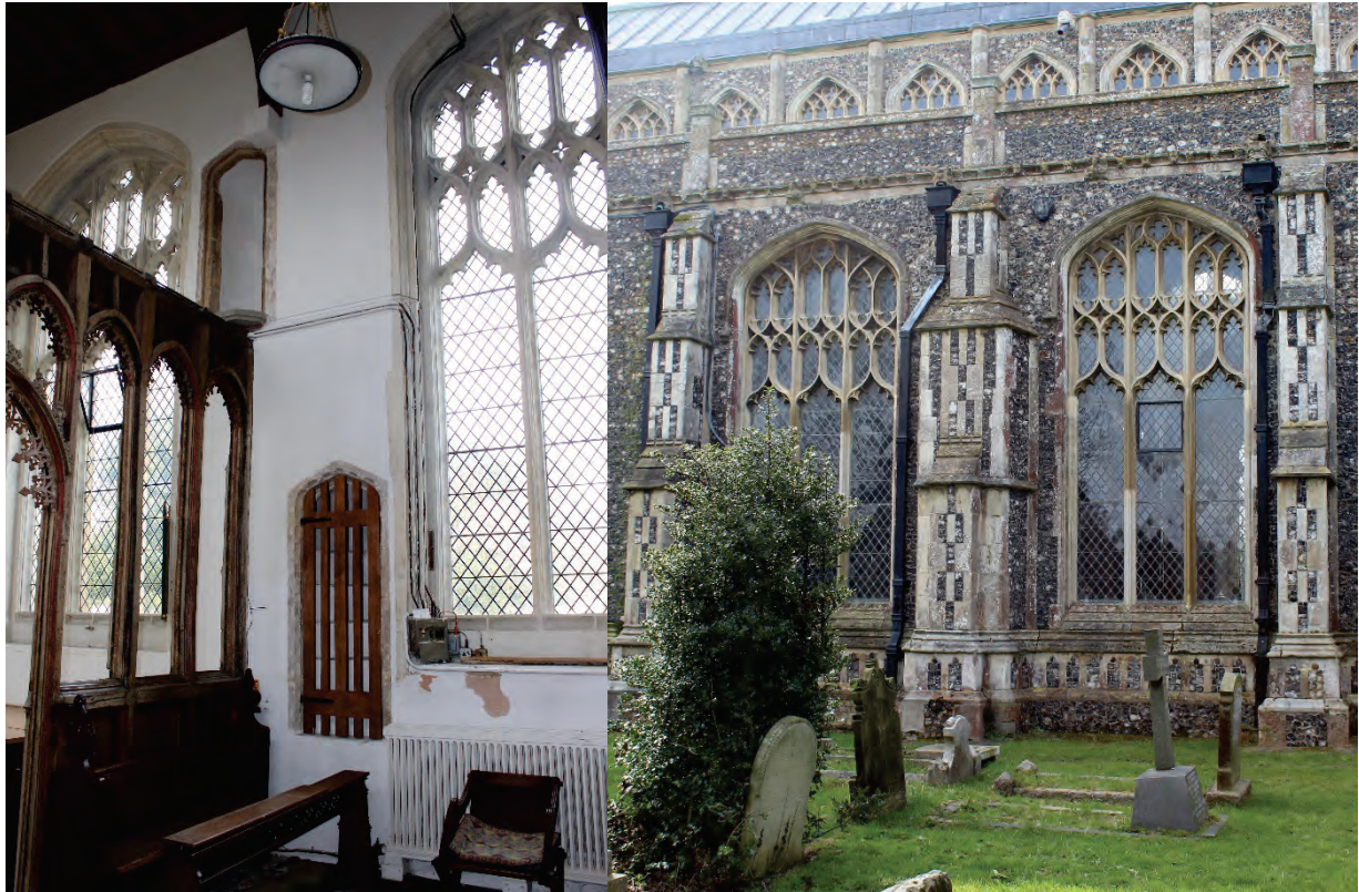
Plate 16. Spiral stairs to a rood screed at St Edmunds church, Southwold. Note how far the of the entrance of the stair is from the floor level and the height achieved in half a turn of the 'vice'(left). Exterior view of the rood stair turret which is hidden within the larger buttress in the centre of the picture (right)
