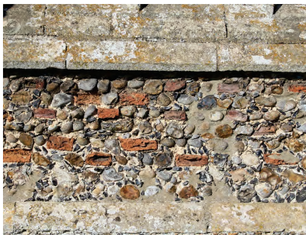
Plate.14. Each element of the church can be characterised by the treatment of its exterior wall face; the south porch (left) uses red brick set amongst in a regular pattern, the north aisle (centre) is composed of large pale flints, and limestone rubble highlighted against black-flint galleting and the chancel (right) uses knapped black flint contrasting with pale limestone dressings
