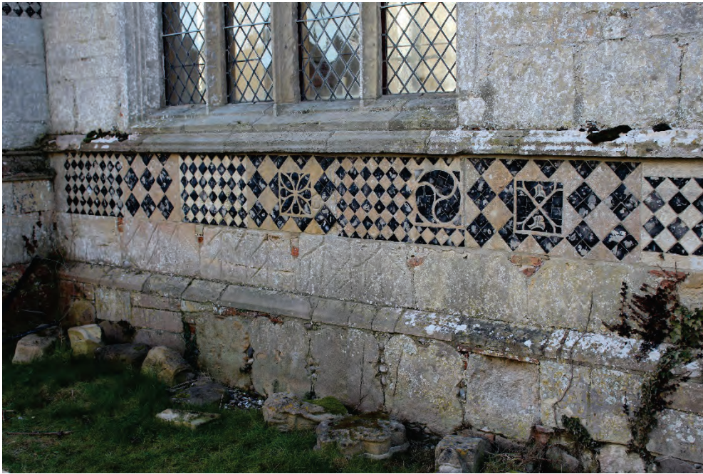
Plate 2. Decorative flushwork panels taken from the parapet and cross-sections of quatrefoil columns that would have once divided the nave from the aisle reused in the church built 1696.
