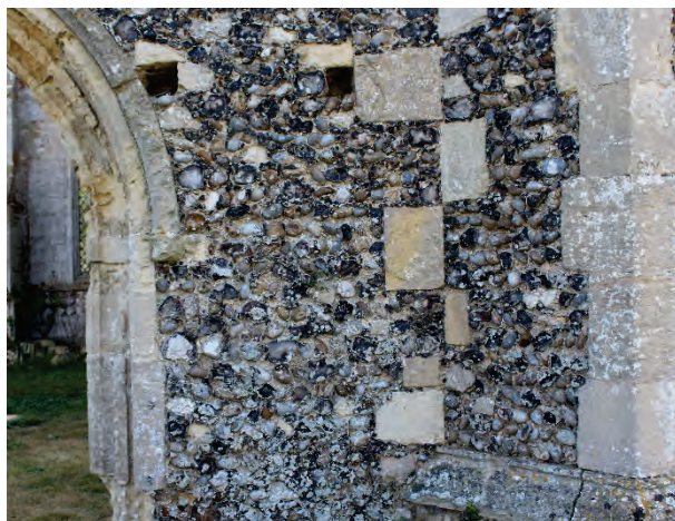
Plate.14. Each element of the church can be characterised by the treatment of its exterior wall face; the south porch (left) uses red brick set amongst in a regular pattern, the north aisle (centre) is composed of large pale flints, and limestone rubble highlighted against black-flint galleting and the chancel (right) uses knapped black flint contrasting with pale limestone dressings
