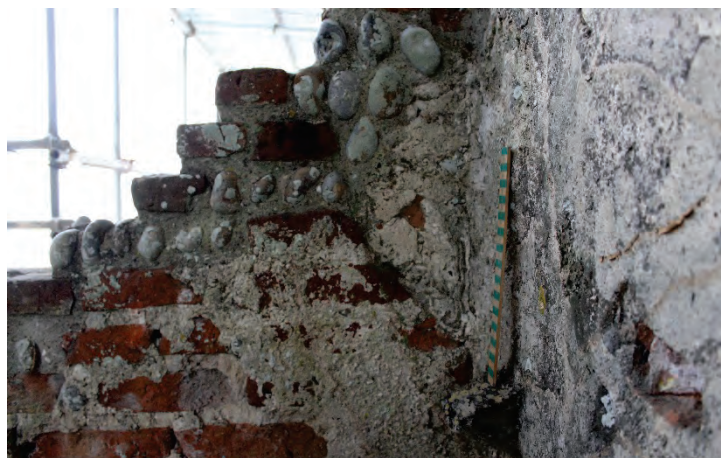
Plate 20. The scale rests on a fragment of projecting limestone stone whilst a curving shape can be seen in the outline of the brickwork of the wall behind
