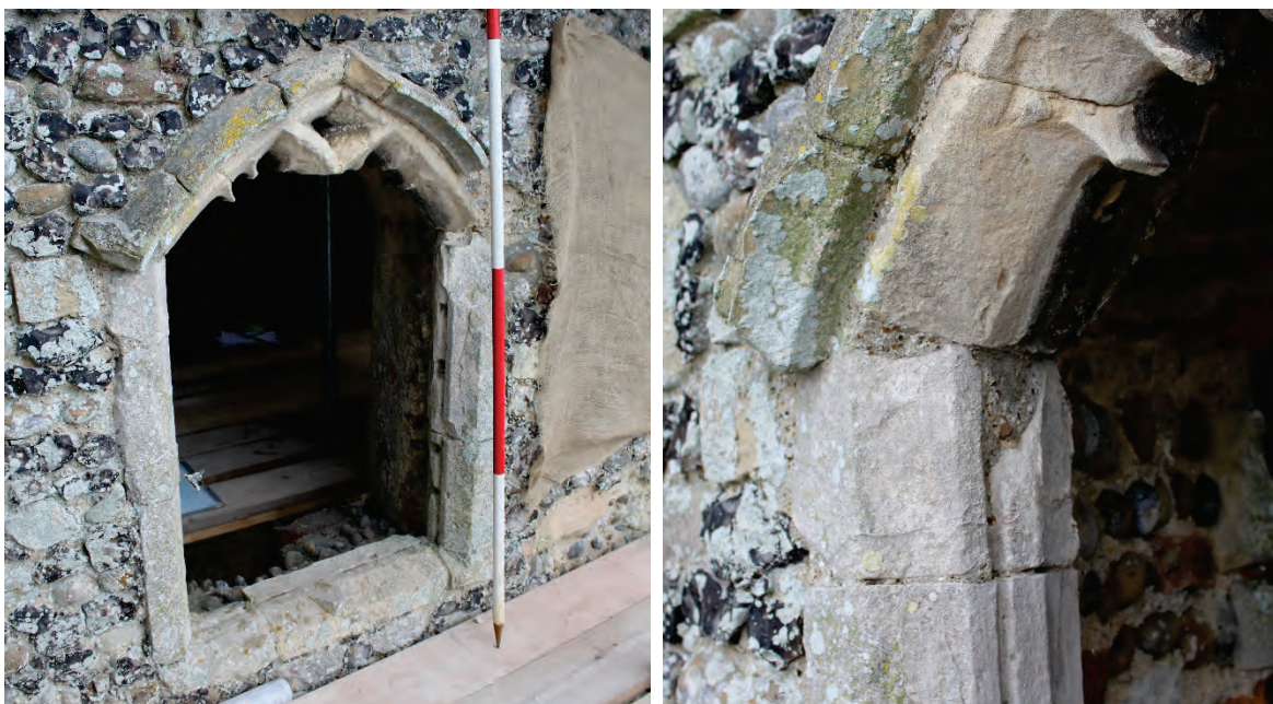
Plate 19. First floor window in the east wall of the north aisle. The tracery in the window head and the hood moulding resembles that used in the clerestory, however the stones here are mis-matched (right) and the hood-moulding too short suggesting that the window has been cobbled together from parts.
