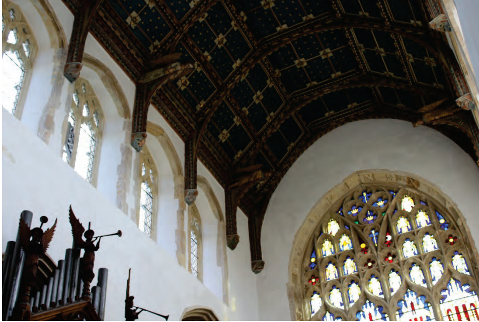
Plate 11. Example of wall posts at the Church of St Edmunds, Southwold
