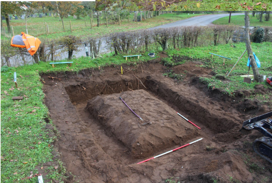
Plate 3 (left). Trench 1 groundworks. The WC was to have a raft foundation measuring 4m x 3m with a deep 'toe' around its perimeter (the slit trench); it was centred in a larger stripped area, measuring 5m x 5m, to enable the construction of timber formwork in which the foundation would be cast.
