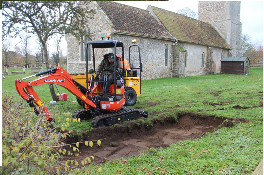
Plate 3 (left). Trench 1 groundworks. The WC was to have a raft foundation measuring 4m x 3m with a deep 'toe' around its perimeter (the slit trench); it was centred in a larger stripped area, measuring 5m x 5m, to enable the construction of timber formwork in which the foundation would be cast.
