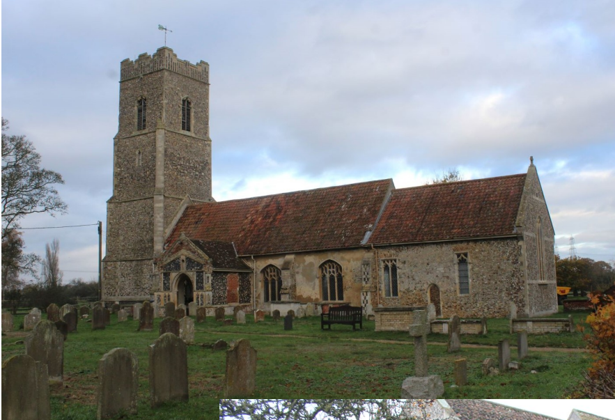
Plate 1 (left) The church of St John the Baptist viewed from the SE. The nave and chancel have 13th century origins, the porch was added in the late 14th and the 'new' tower added in the mid-15th centuries. The church is set back from the road within a large churchyard set out predominantly to the south
